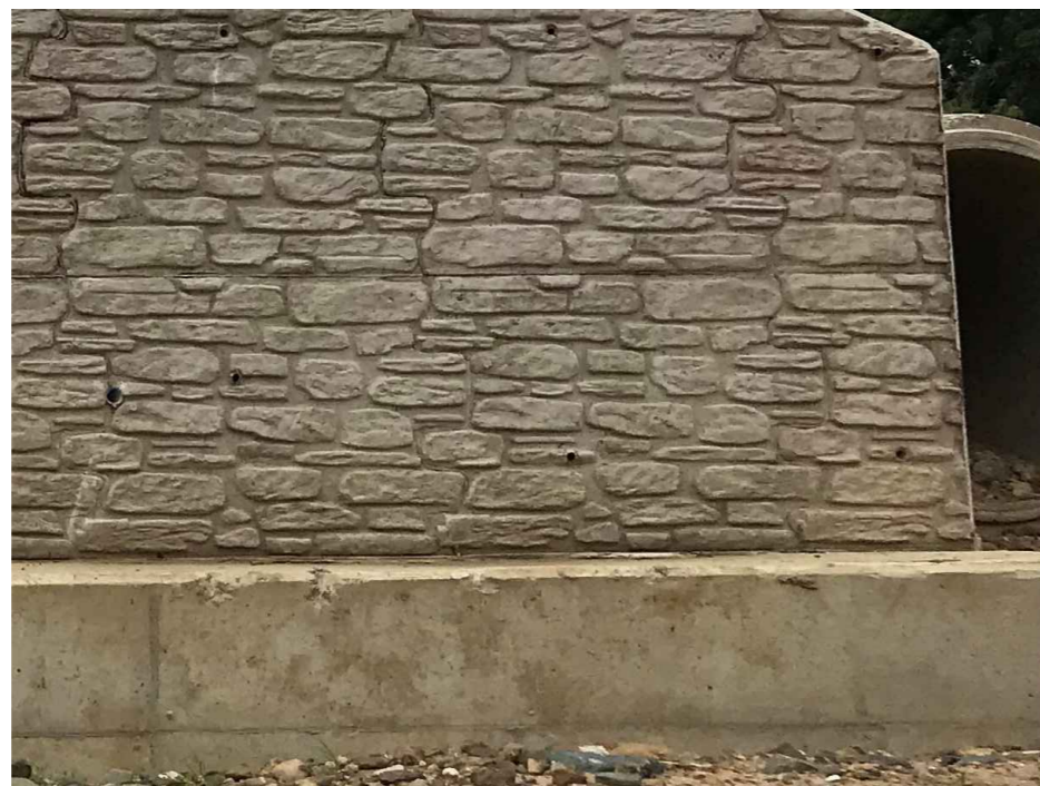
ROCK FINISH DETAIL (WINGWALLS ONLY)
