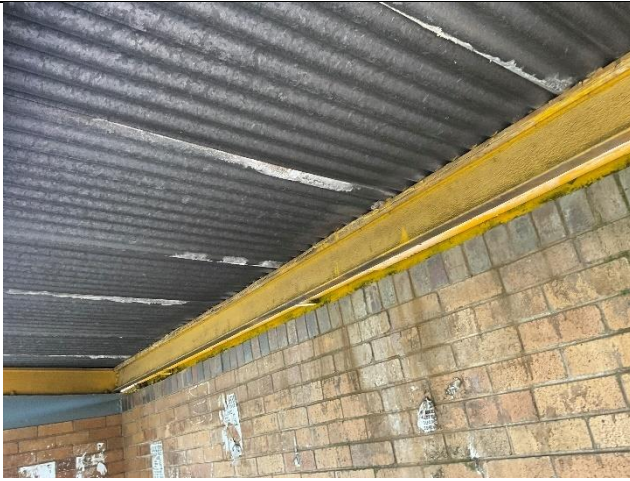
Figure S13: Platform Shelters – white rust as surface zink observed on aluminium roof sheeting
