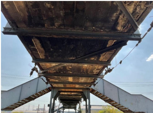
Figure S15: Bridges - fire damages on steel members and precast concrete slabs
