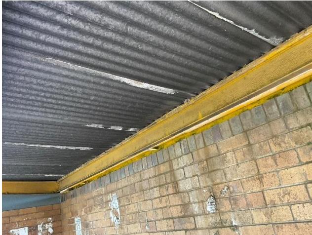
Figure S13: Platform Shelters – white rust as surface zinc observed on aluminium roof sheeting
