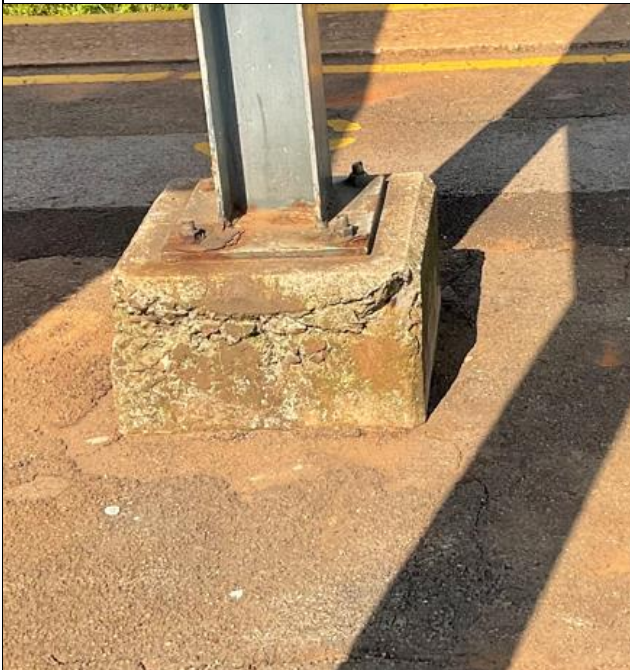
Figure S19: Bridges Supports – Cracked concrete plinths
