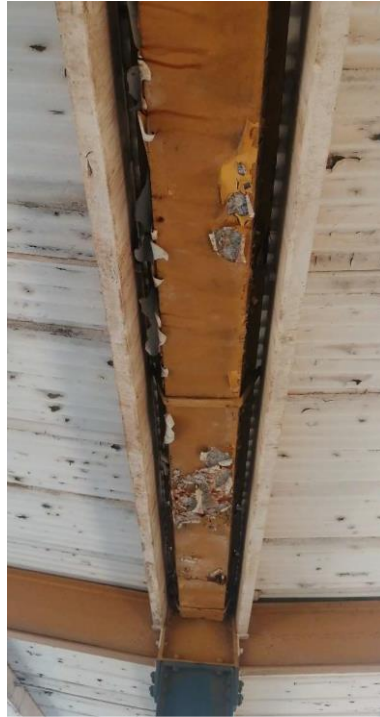
Rusted members and gutters on shelter
