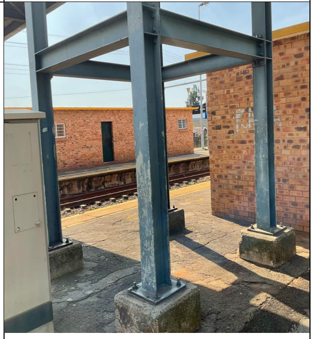
Figure S20: Bridges column supports – Concrete plinths and steel columns are structurally sound
