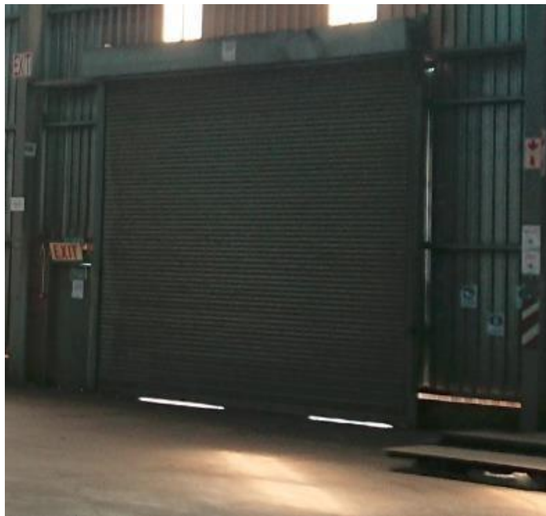
Figure 3: Gap under Roller Door
