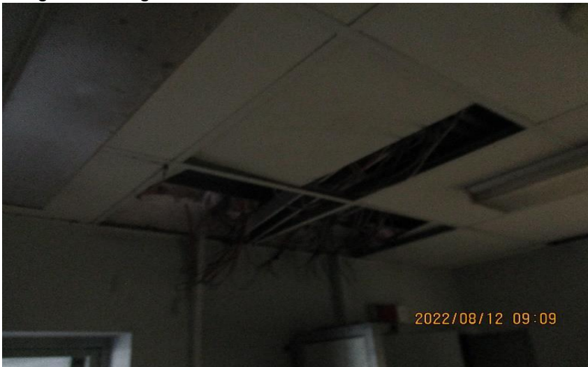
Image 3: Ceiling at Ticket Office
