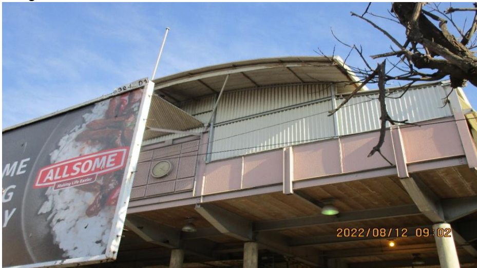
Image 5: External Steel Structure
