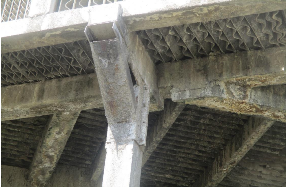
Photo 4: Rusted stainless steel knee-bracing -type A
