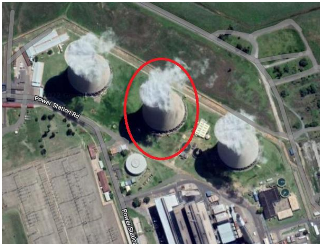
Figure 1: Plant layout illustrating Cooling Tower 2
