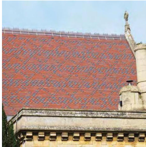
Above: Ornamental tiles in red blue blend and Staffordshire blue were used to recreate the polychromatic diaper pattern on this Gothic Revival church.
