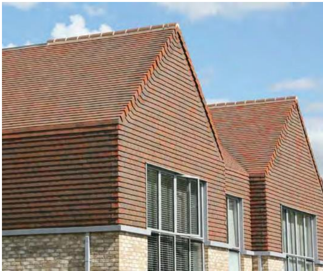
Above: New homes at Audley's Chalfont Dene luxury retirement village use country brown sanded tiles with half round ridges, valley tiles and bonnet hips.
