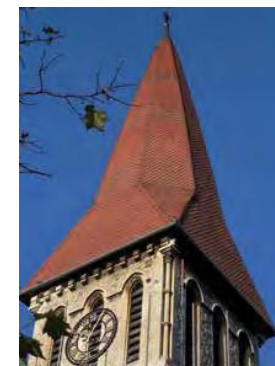
Above: St John The Evangelist Church Dulwich, plum red with bands of country brown tiles in a mix of club and fishtail ornamental tiles, together with purpose-made hips.
