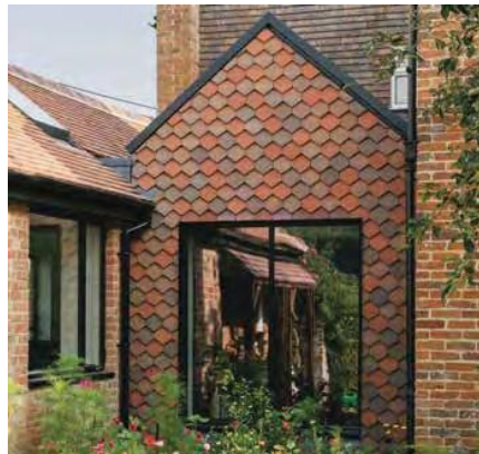
Above: A mixed blend of Dreadnought handmade deep red, bronze and purple brown arrowhead tiles clad a modern extension to a historic building.
