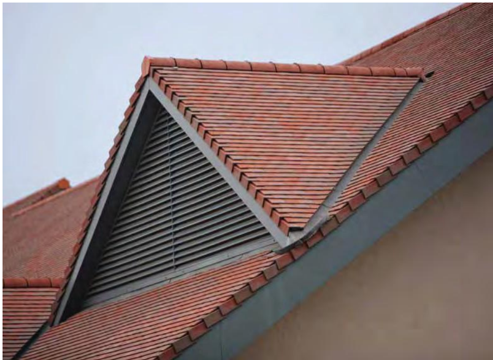
Top: Dreadnought's red blue tiles on Moseley Hospital. The use of cloaked verges and half round ridges as a "dry fix" produces a neat finish.
