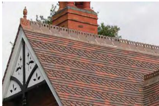
Above: This Victorian house was re-roofed using a mixture of brown brindle and country brown tiles with ornamental club tiles to match the original. Ornamental finials and ridge tiles were hand-made to match the originals.
