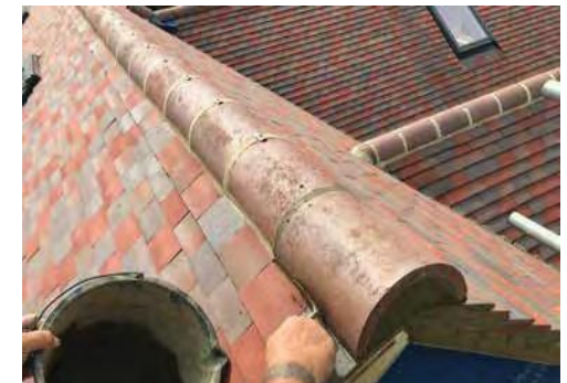
Above: A mechanically fixed mortar bedded ridge
