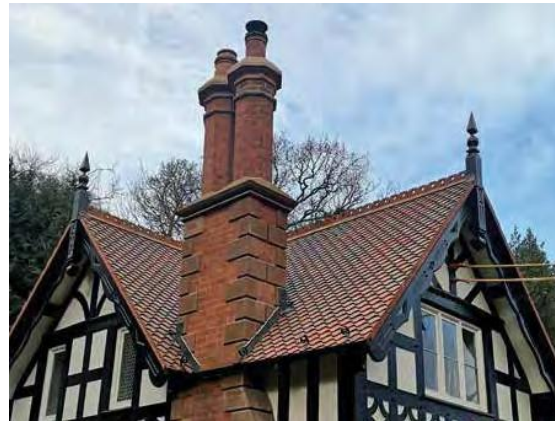
Above: Dreadnought's brown antique clay roof tiles were used to sympathetically restore the roof on the Grade II listed Engine Room at Walthamstow Wetlands in East London
