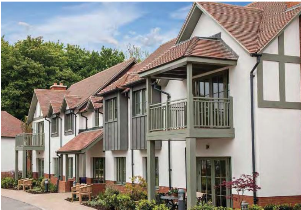
Above: New homes at Audley's Chalfont Dene luxury retirement village use country brown sanded tiles with half round ridges, valley tiles and bonnet hips.
