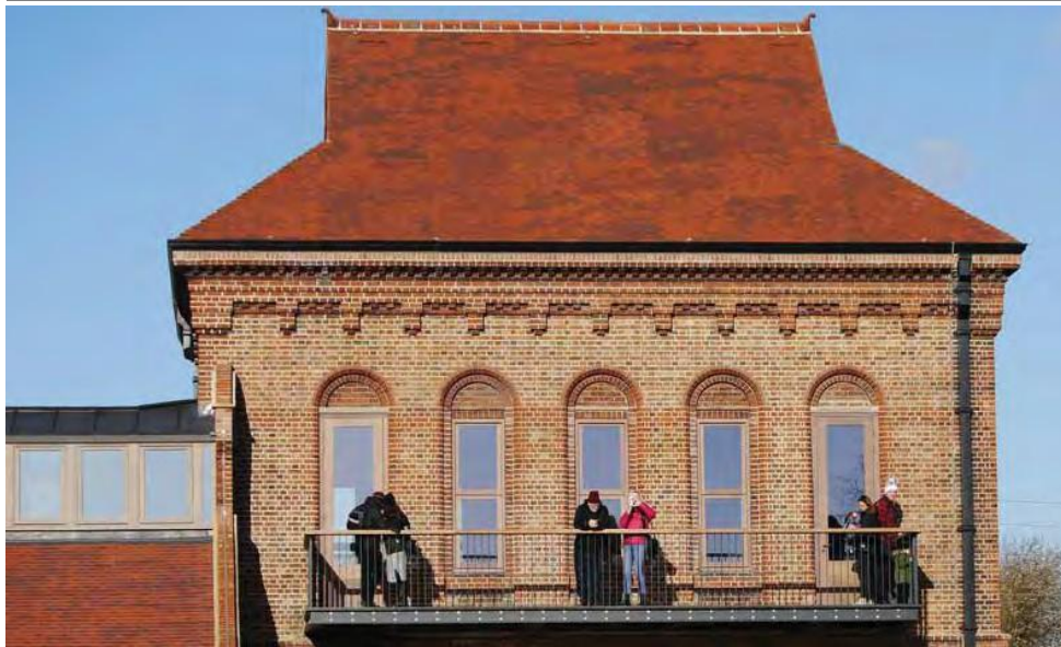
Above: Dreadnought's brown antique clay roof tiles were used to sympathetically restore the roof on the Grade II listed Engine Room at Walthamstow Wetlands in East London
