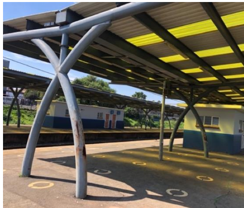
4. Faded paint on steel structures
