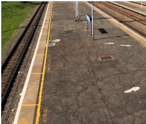
3. Cracked platform floor surface.
