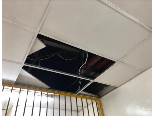
2. Damaged ceiling in ticket office
