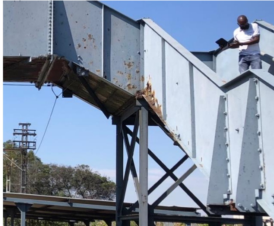
8. Corrosion on platform bridge
