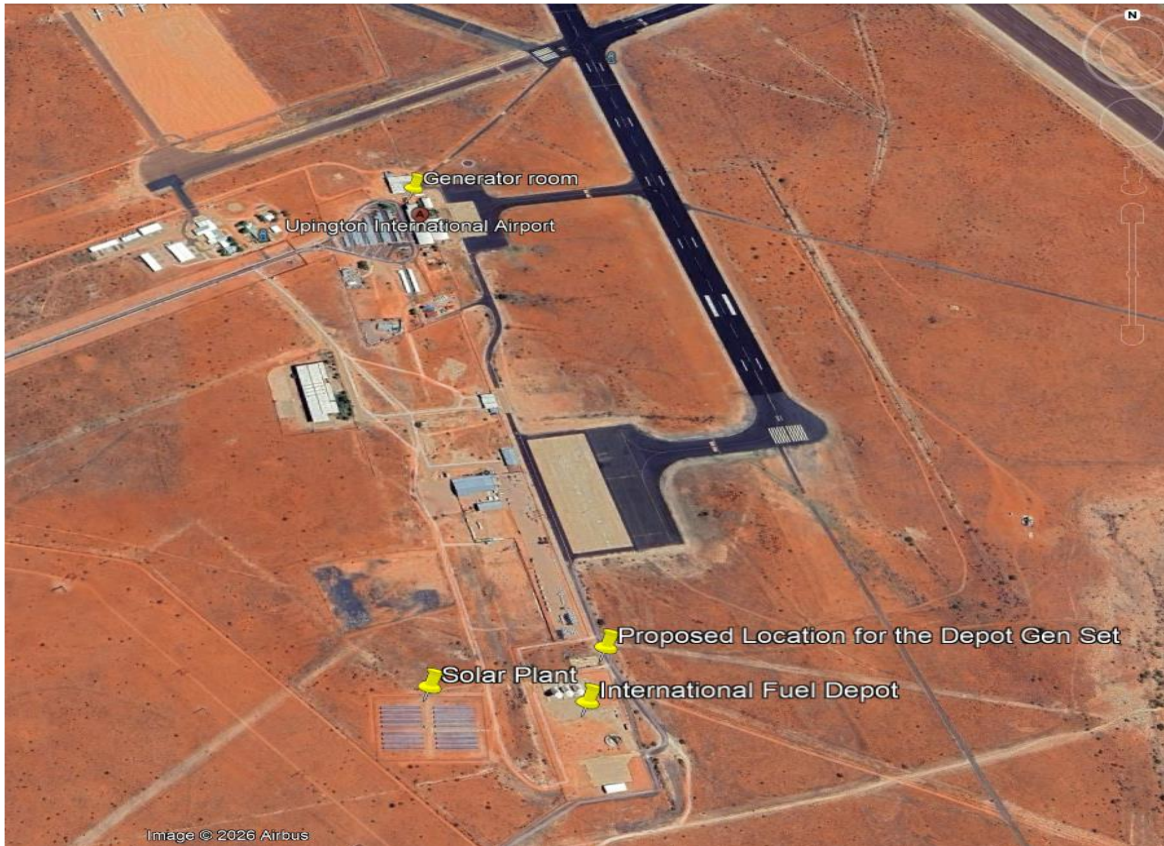
Figure C4.1A: UPN Aerial View Image
