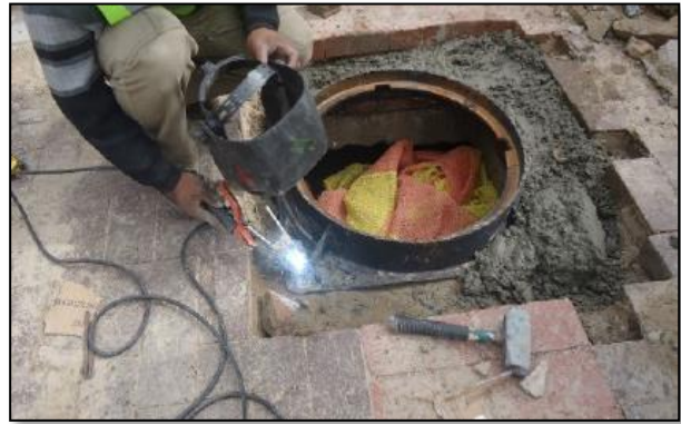
Fig. 17 Welding the frame in place
