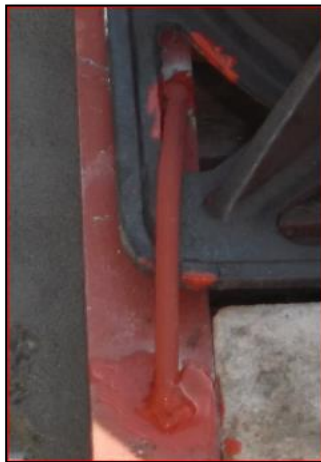
Fig. 15 Angle-irons used to attach the frame to the I-Beam
