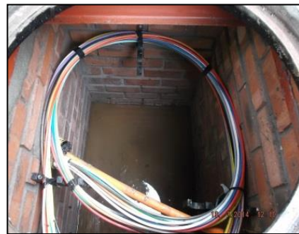
Fig. 24 Correct installation of tube slack
