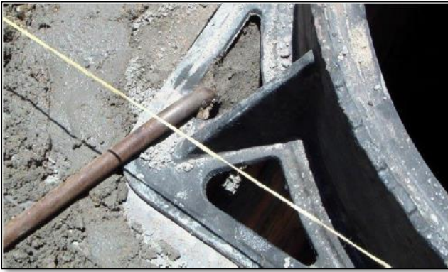
Fig. 16 Attaching the frame
