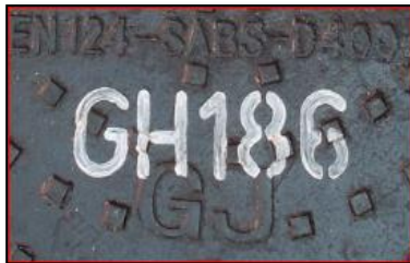
Fig. 25 Manhole number painted on cover
