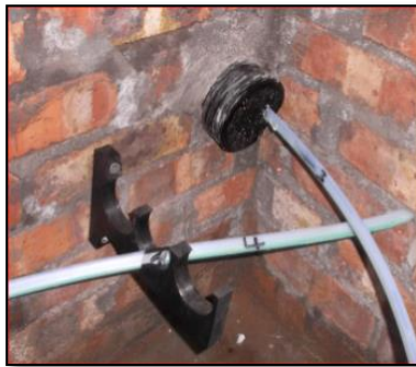
Fig. 23 Brackets and duct spacing (example)
