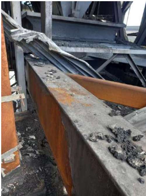
Figure 8: Typical surface corrosion spots
