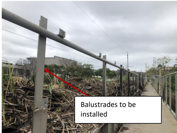
Photo 12: Balustrades to be installed on the pedestrian bridge.
