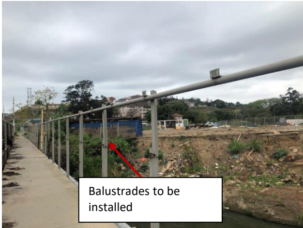
Photo 11: Balustrades to be installed on the pedestrian bridge.
