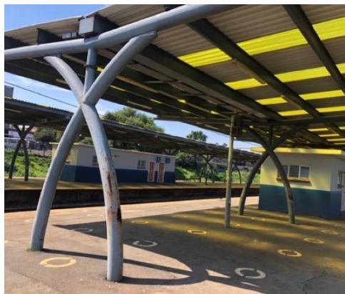
4. Faded paint on steel structures
