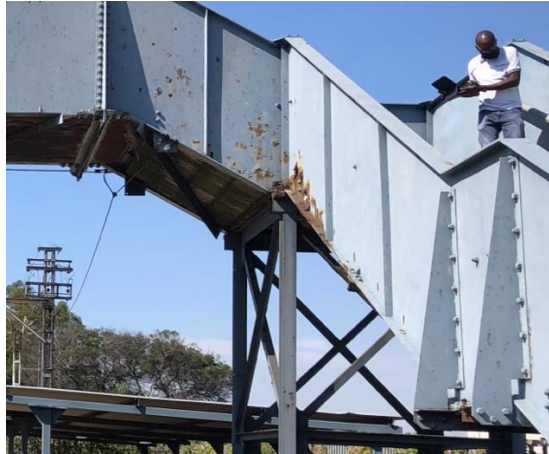
8. Corrosion on platform bridge
