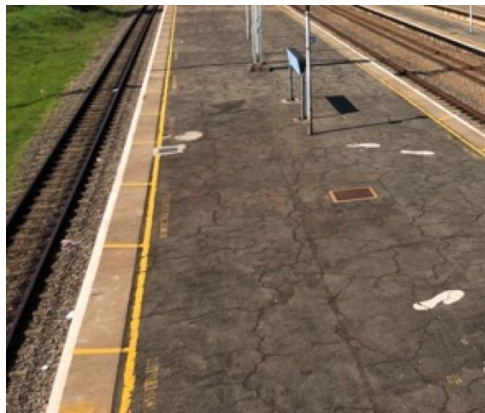
3. Cracked platform floor surface.
