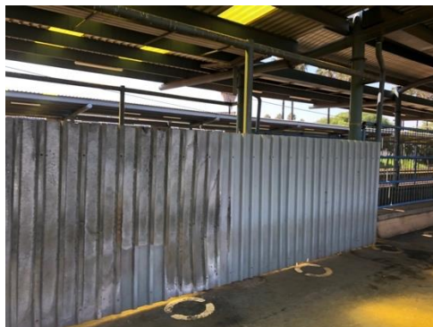
4. Faded paint on steel structures
