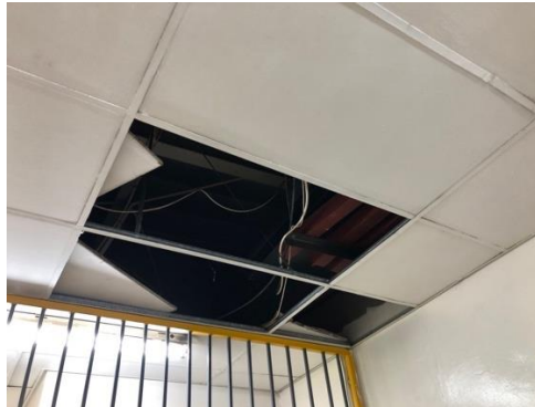
2. Damaged ceiling in ticket office
