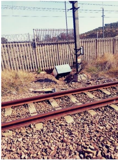
Figure 1: Shows under-dig breach
