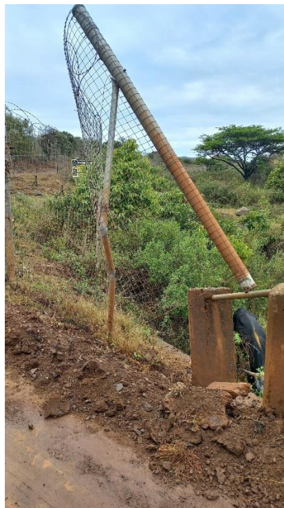
End of fencing repair on left bank. Total repair =57m on right bank, includes new fencing, y-standards, foundation and poles.
