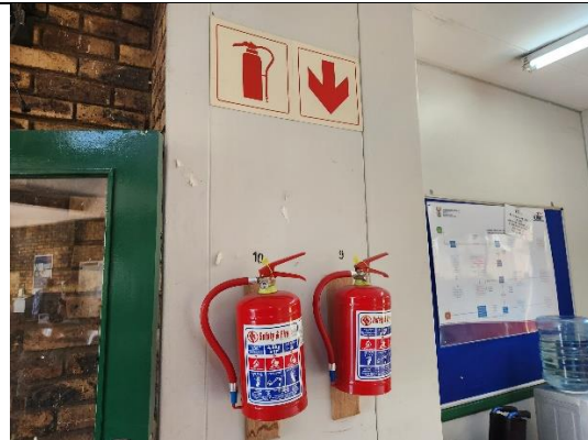
Figure 8: Portable fire extinguisher with fire signage in fair working condition
