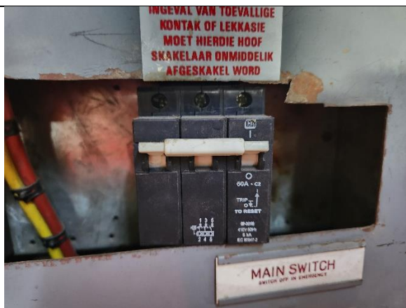
Figure 41: Distribution board with missing covers and exposed wiring
