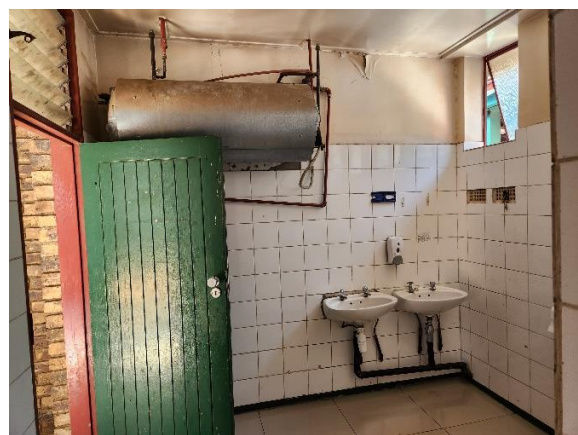
Figure 6: Wall mounted external high-pressure geyser in fair working condition
