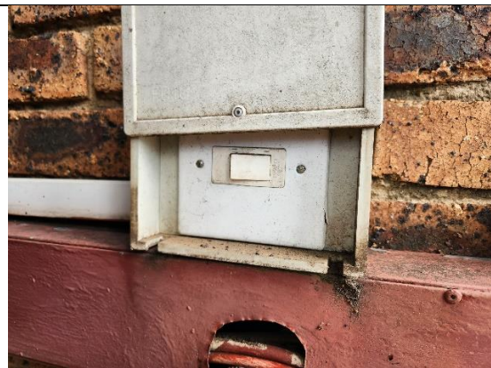
Figure 14: AC Isolator in fair working condition
