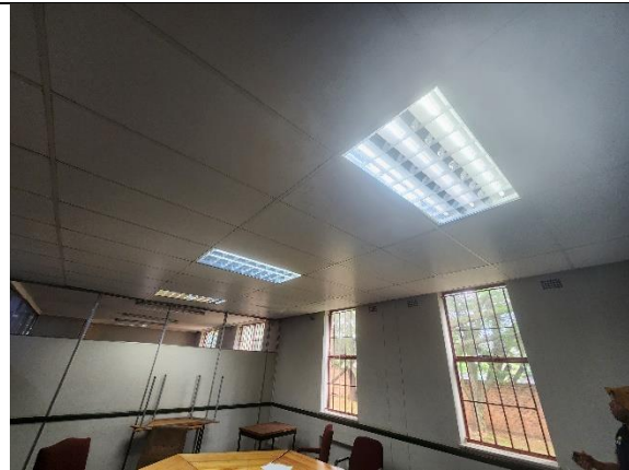
Figure 32: Recessed light fittings in fair working condition
