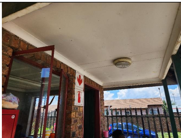
Figure 23: Old bulkhead to be replaced with energy saver type
