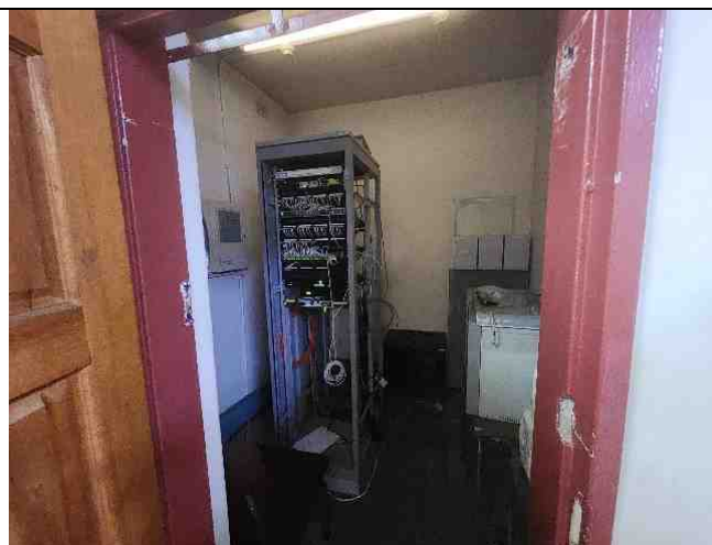
Sever Room – Inadequate Fire Suppression system
