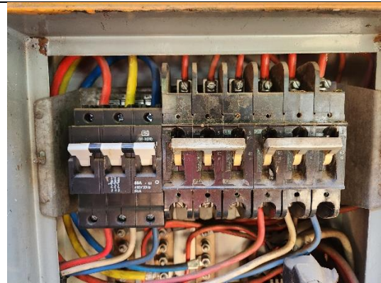
Figure 8: Main electrical distribution board with old switch gear
