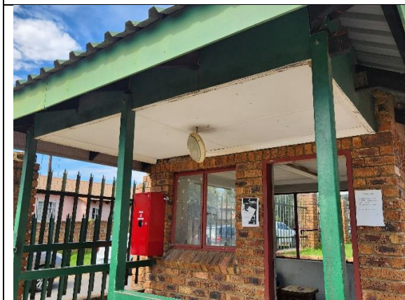
Figure 11: Old bulkhead fitting hanging by wiring
