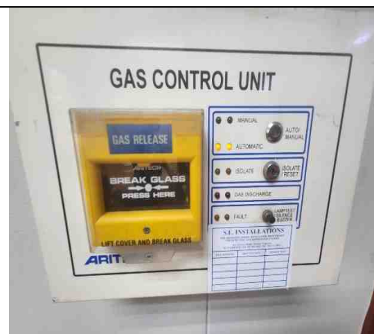
Fire Suppression system with no service dates
