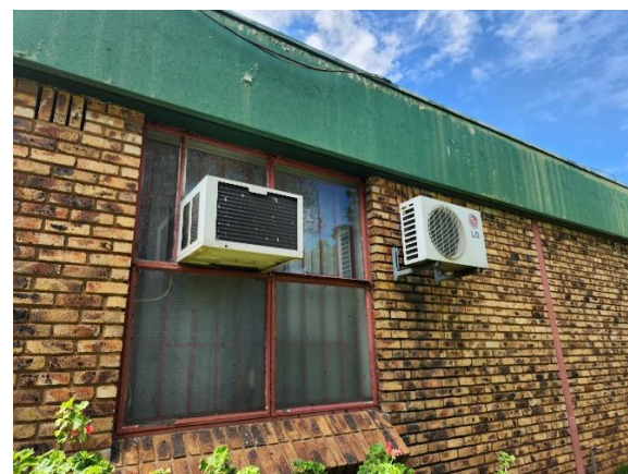
Figure 5: Outdoor and window console air conditioning units in fair to poor working condition
