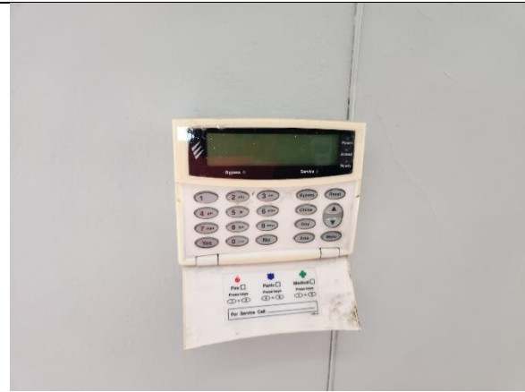
Figure 38: Burglar alarm keypad
