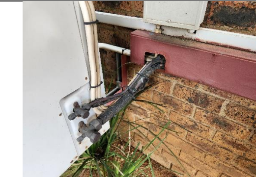
Figure 4: Outdoor air conditioning unit refrigeration pipe in poor working condition
