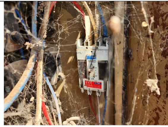
Figure 4: Main Circuit Breaker, 150A
