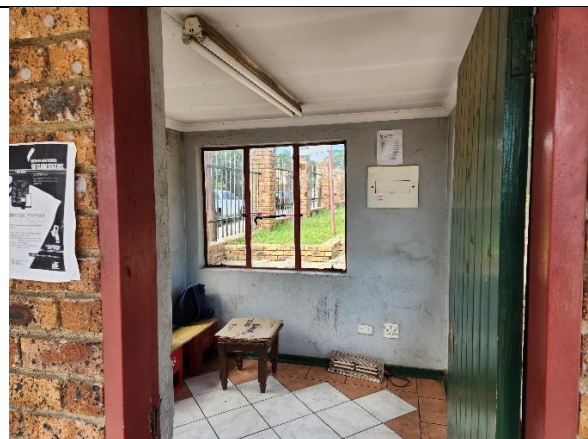
Figure 12: Old surface mounted open channel fitting to be replaced with weatherproof type
