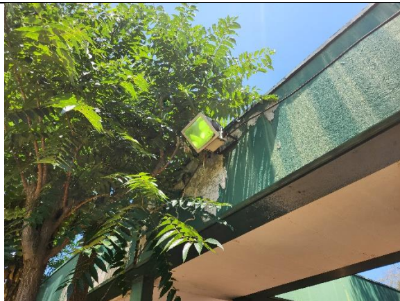
Figure 33: Security flood light in fair working condition with poor wiring installation
