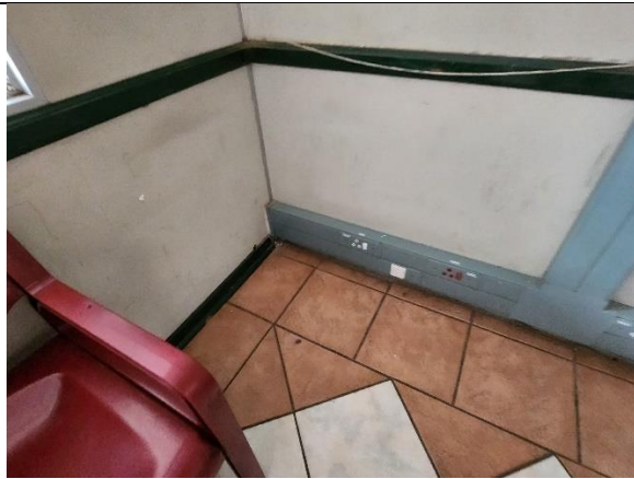
Figure 37: Power supply wiring to be run inside conduit / powerskirting
