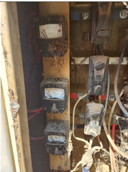
Figure 5: Kiosk with old switch gear and meters
