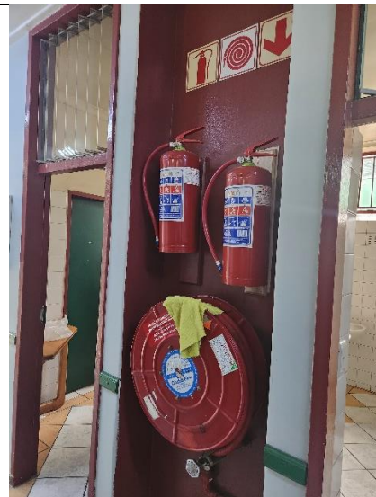
Figure 10: Firefighting equipment in fair working condition with proper signage
