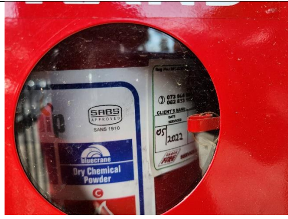
Figure 2: Portable fire extinguisher equipment due for overdue for service
