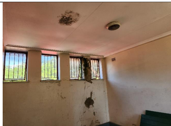
Figure 18: Old bulkhead fitting to be replaced
