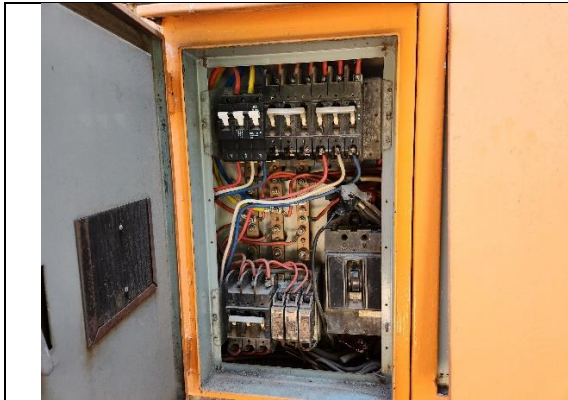
Figure 7: Main electrical distribution board with old switch gear
