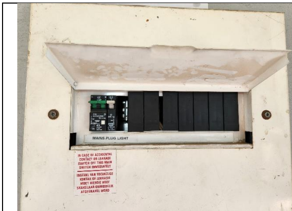
Figure 13: Guardhouse DB in fair working condition
