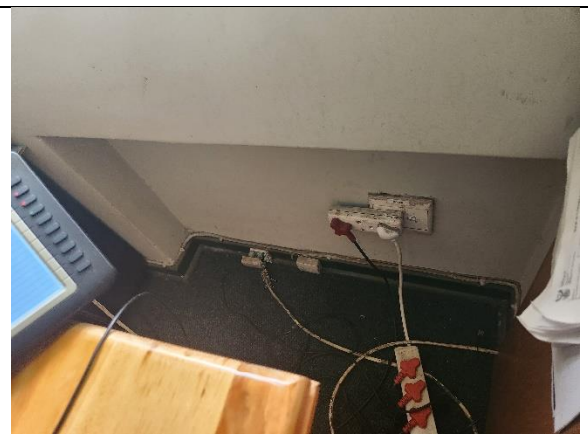
Figure 24: Additional SSO's required in offices
