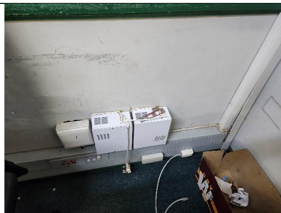
Figure 36: Burglar alarm power point disconnected
