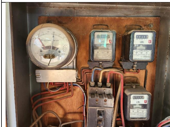
Figure 7: Main electrical distribution board with old switch gear
