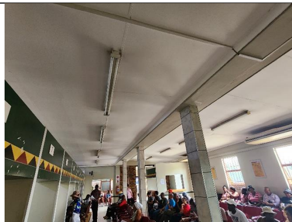
Figure 30: Old open channel light fittings to be replaced with energy saver type fitting
