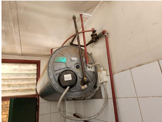
Figure 7: External mounted geyser pipe reticulation in fair work condition
