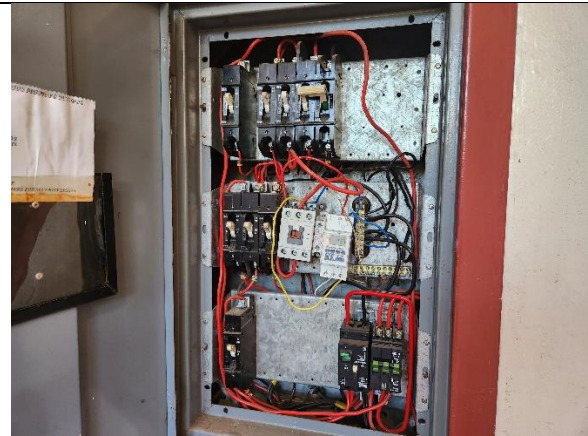
Figure 20: Distribution board in poor working condition. Cover missing and wiring not neat
