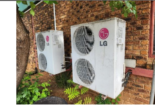
Figure 3: Outdoor air conditioning unit in fair working condition
