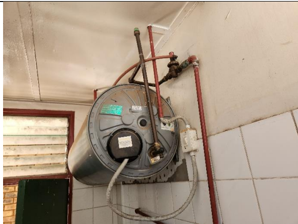
Figure 19: External isolator for geyser in fair working condition
