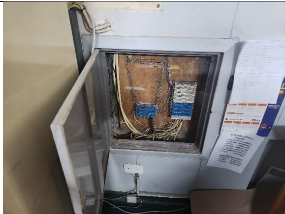
Figure 25: Old Telkom switchboard
