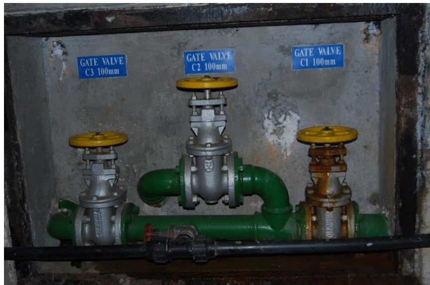
Recess in the gallery control room with Ø100mm back fill lines and valves
