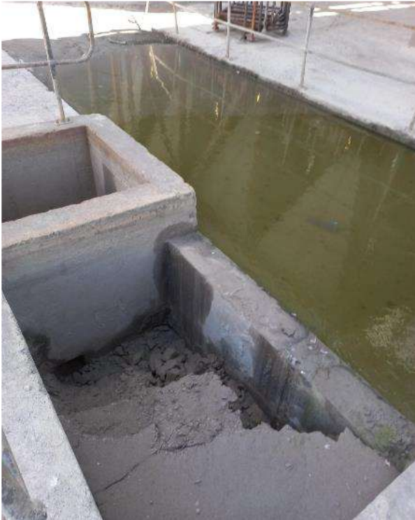
Figure 4: Layout of Ash Recovery Silt Trap
