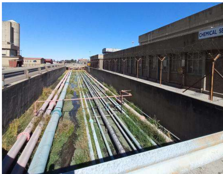
Figure 9: Pipe Trenches
