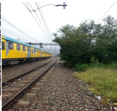
Fig 2.2: Trees encroaching on railway lines
