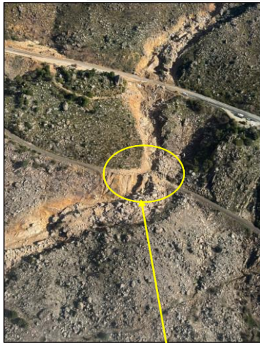
Washaway Point: Track covered in mud and rocks
