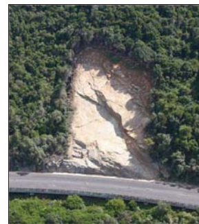
Kaaimans Pass: Failure #2 site Dip slope translational type failure. [M Mohlalane, BKS]
