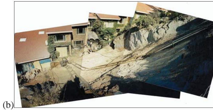
Figure 17 (a) Graphic showing thick quartzite blocks which had slid on a gently wavy, phyllitic, bedding plane daylighting in the slope face. (Bruma Lake, Johannesburg: February 2000). (b) Image taken during post slope clearing inspection: August 2000.
