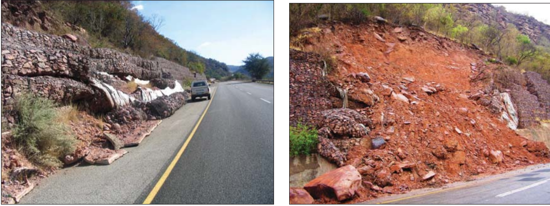
Figure 15 Graphic showing that poor design or maintenance of gabions can lead to recurring public fund expenditures. The images portray a slope remediation effort that was in fact a poor mitigation approach. (Limpopo Province, April 2008: Highway R518 (left and right))
