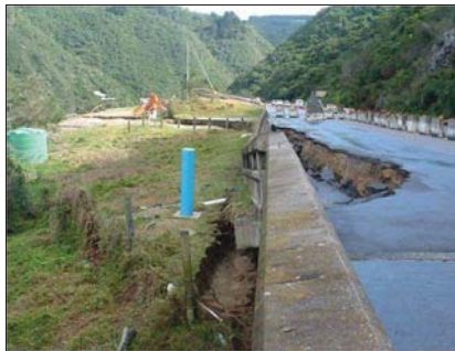
Kaaimans Pass: August 2006: Failure #1 site Highway, house at left and railway below affected. [M Mohlalane, BKS]
