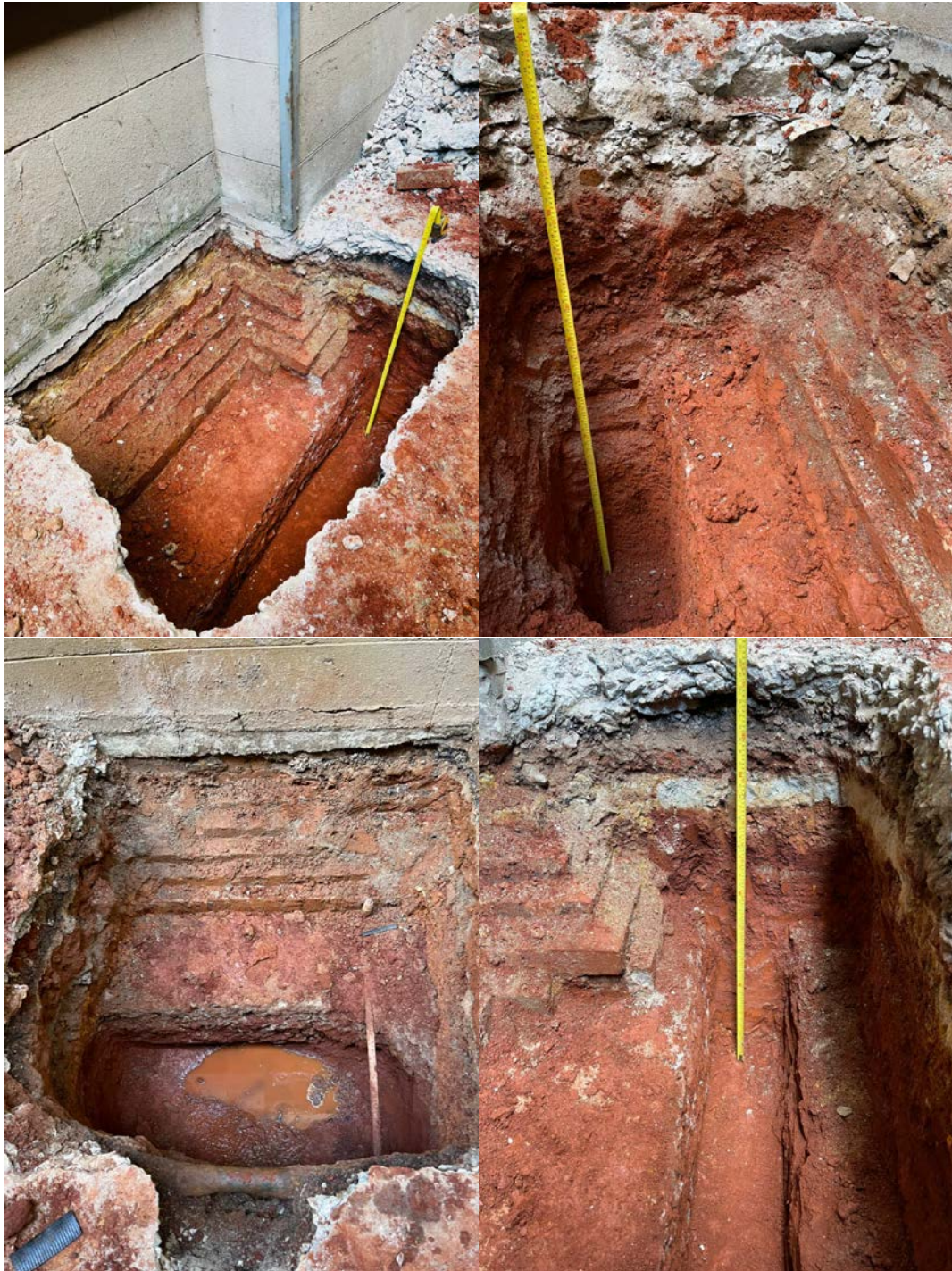
Figure 5: Shows the typical excavated test pits during the site investigation
