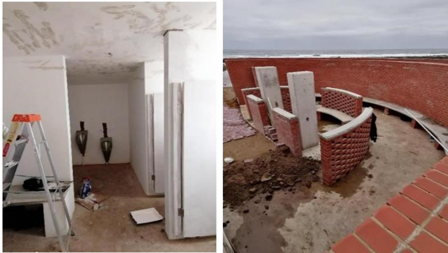
Selection of pictures showing some unfinished works on building G and H. They include uncleaned brickwork and concrete edges, unfinished soffits, floors, and other fittings including external shower fittings.
