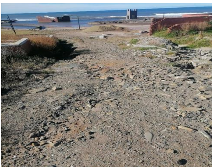
Ramp work needs to be completed in full – layer works, compaction and actual finish and retention structure.
