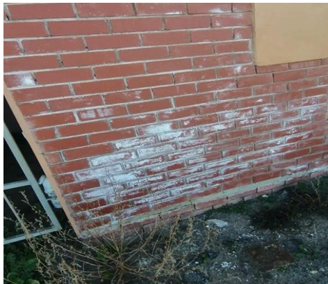
Efflorescence needs to be dealt with in a major way on all face brick surfaces. Potentially the contractor should factor in sealing face brick walls.
