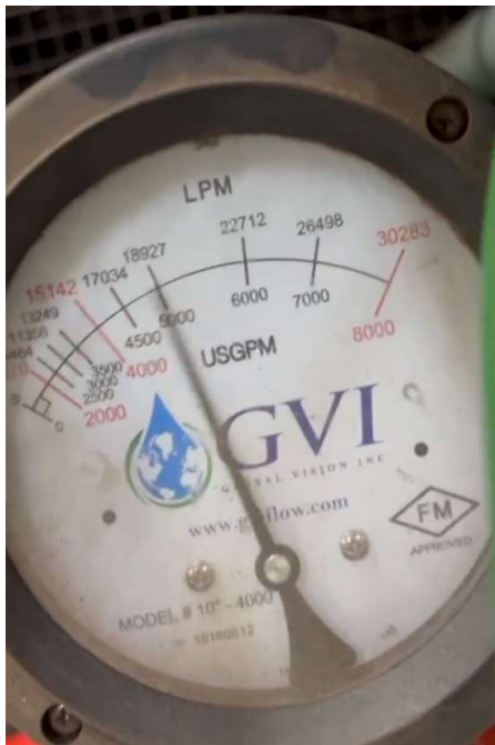
NEW ENGINE PUMPSET DELIVERING REQUIRED FLOW
