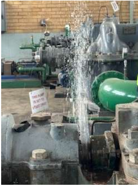
TYPICAL PUMP LEAKS
