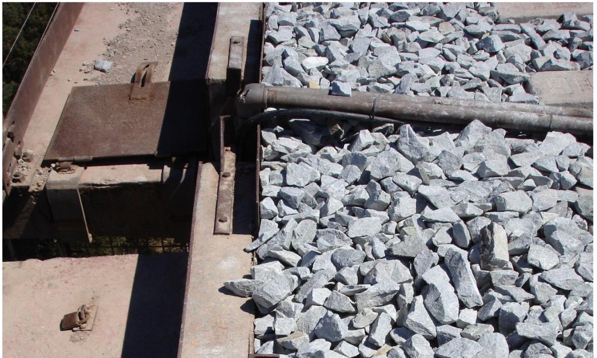
Appendix B Figure 6: Expansion joint on the Sishen side of the ORB by the right hand side – It is used as the entrance to the hardware of the monitoring system
