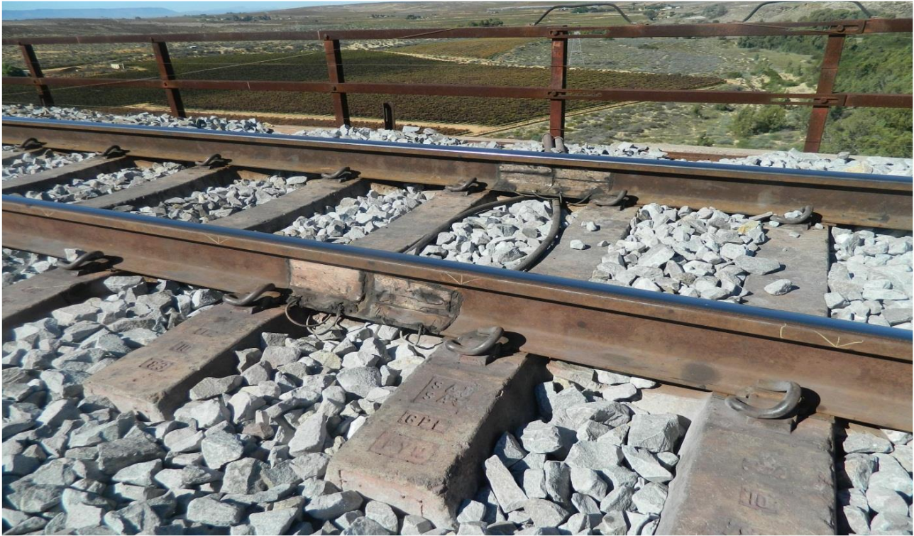
Appendix B Figure 10: Rail stress and temperature measurements sensors at expansion joint 1 for system 1 and 2
