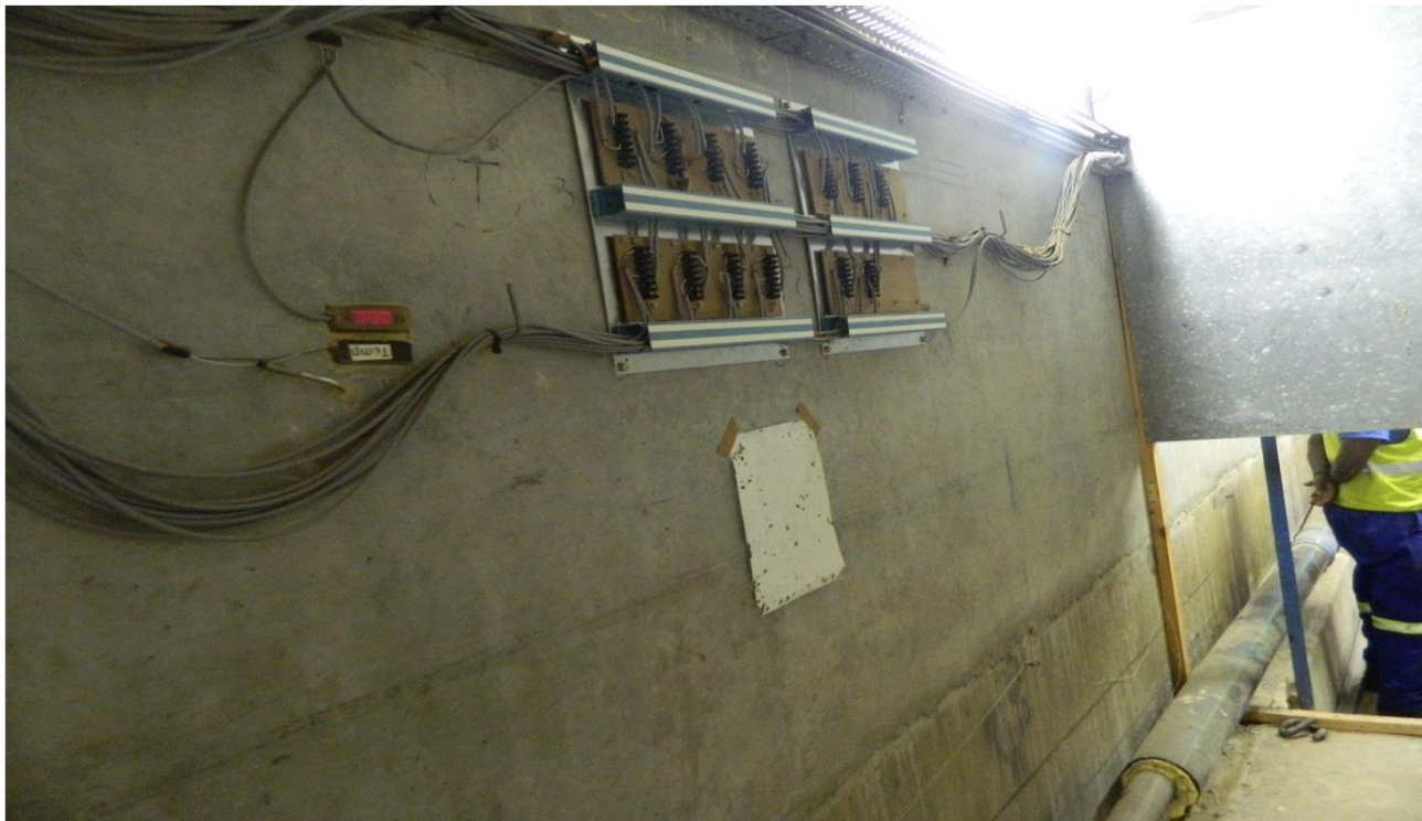
Appendix B Figure 21: Interface connection of system 2 mounted on the left hand side of the hollow deck walls
