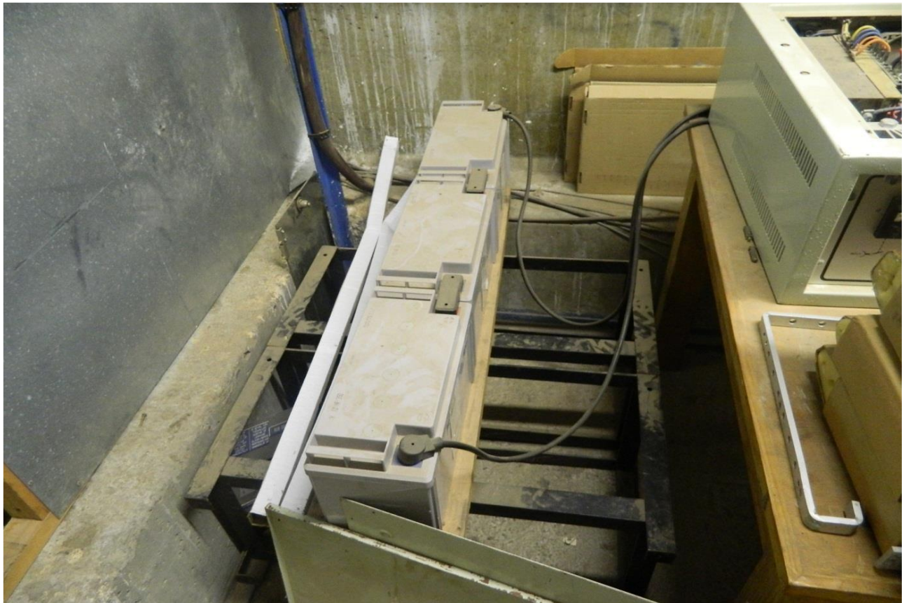
Appendix B Figure 29: Batteries for the uninterruptible power supply of the monitoring system
