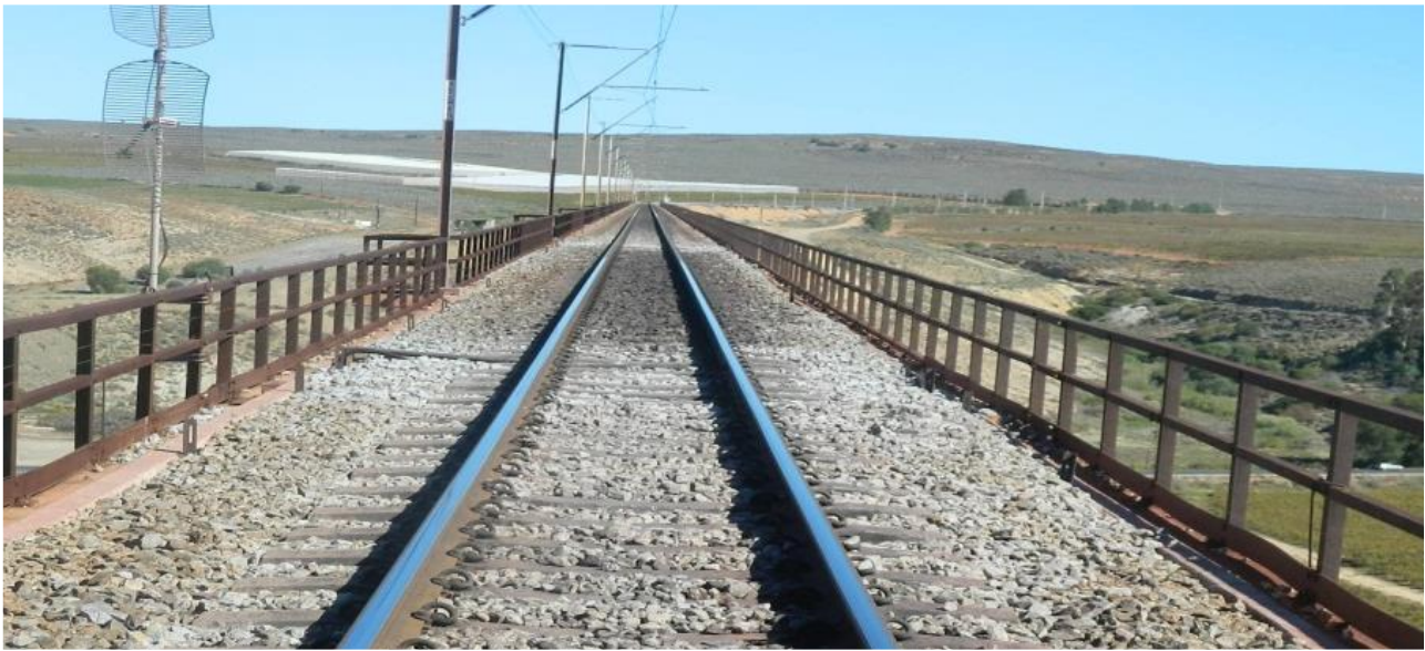
Appendix B Figure 8: Positions of the measurements locations on the Olifants River Bridge indicated by the white ballast at expansion joint 1 (Sishen deck) and expansion joint 2 (Saldanha deck)
