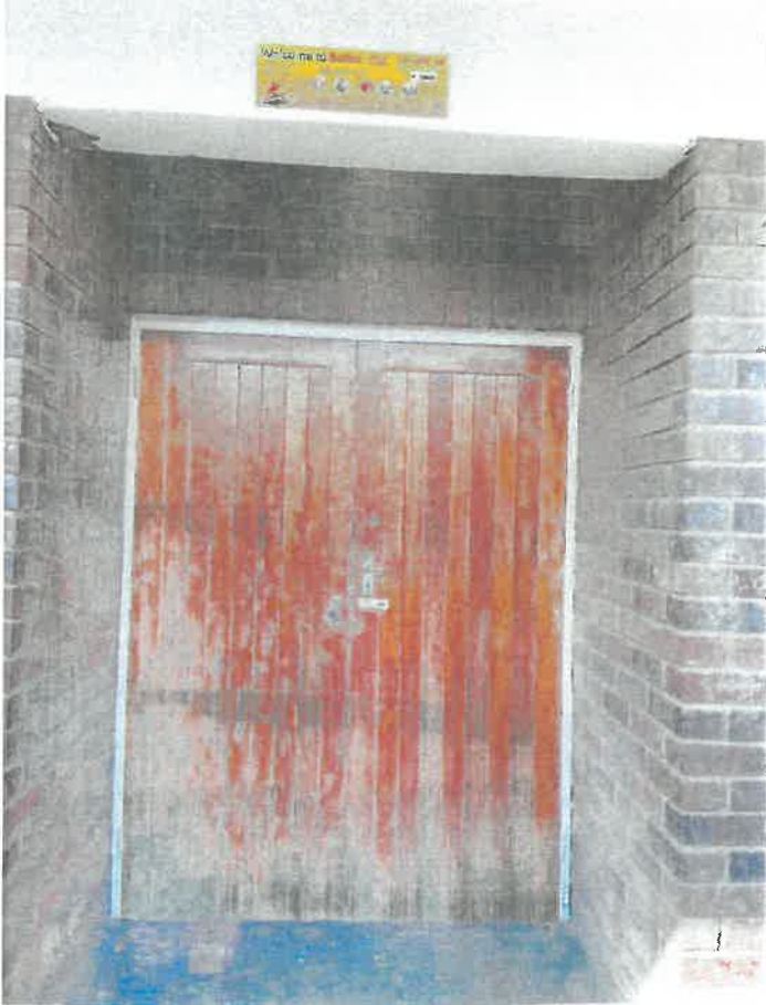
Main door Room 26
