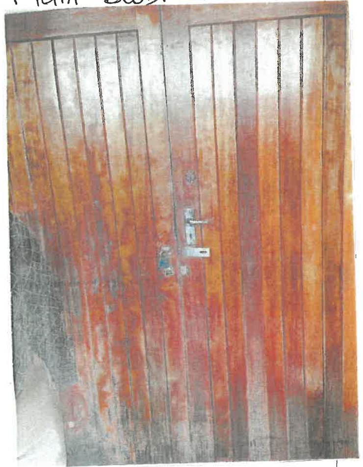
Main door room 26
