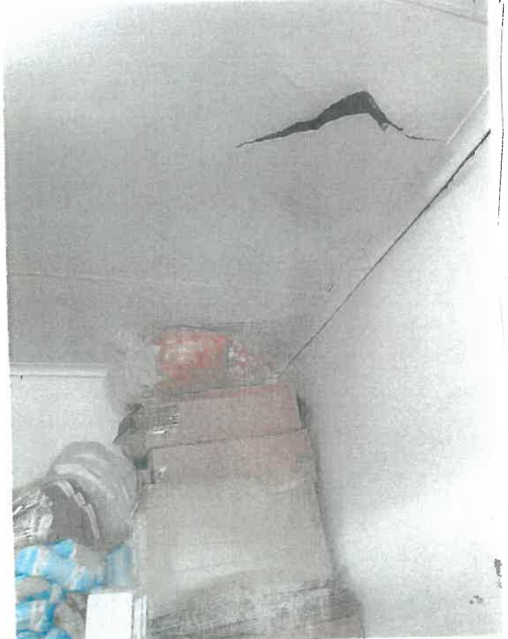
Store room in Room 41
