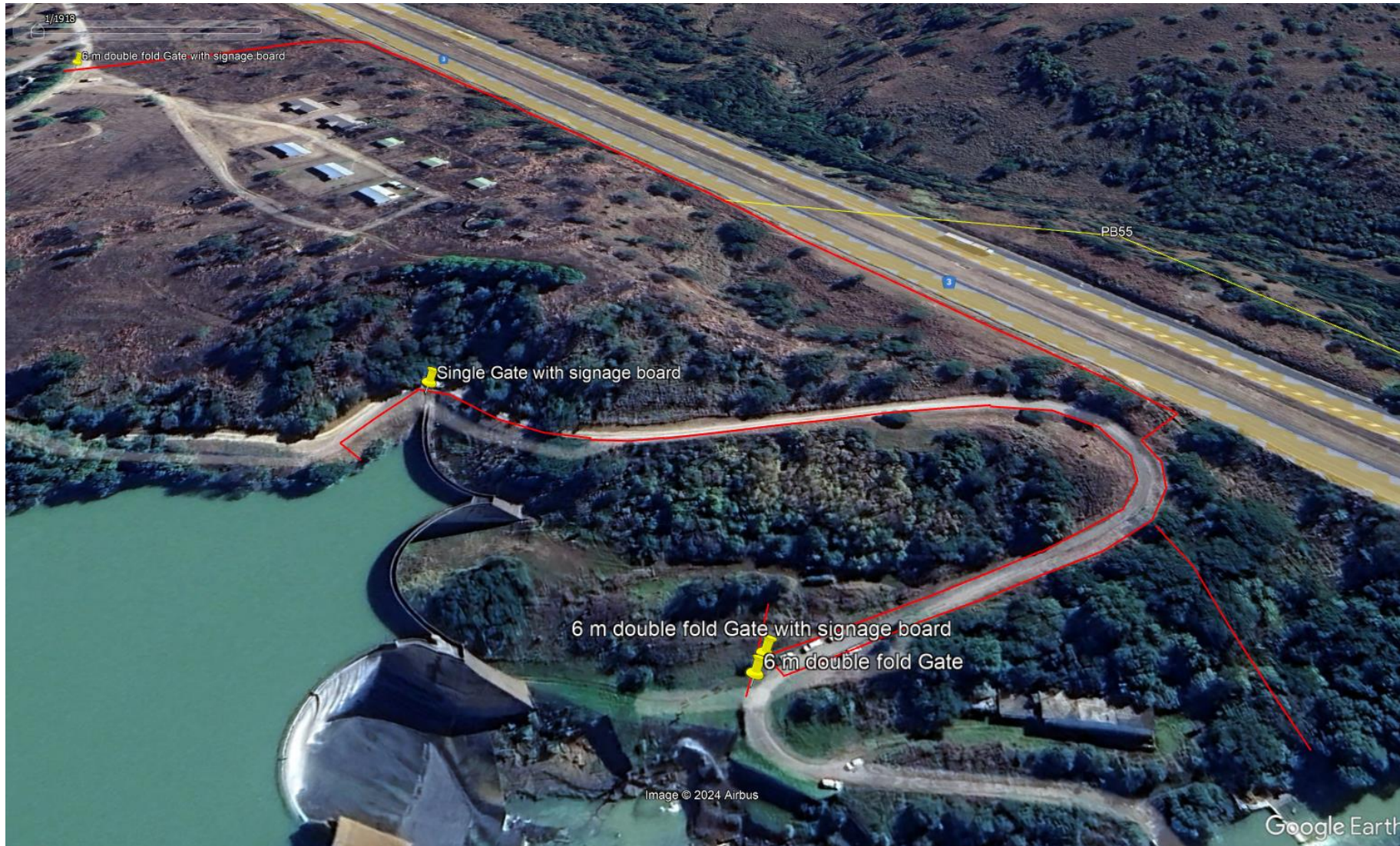
Wagendrift Dam left bank fence line in red
