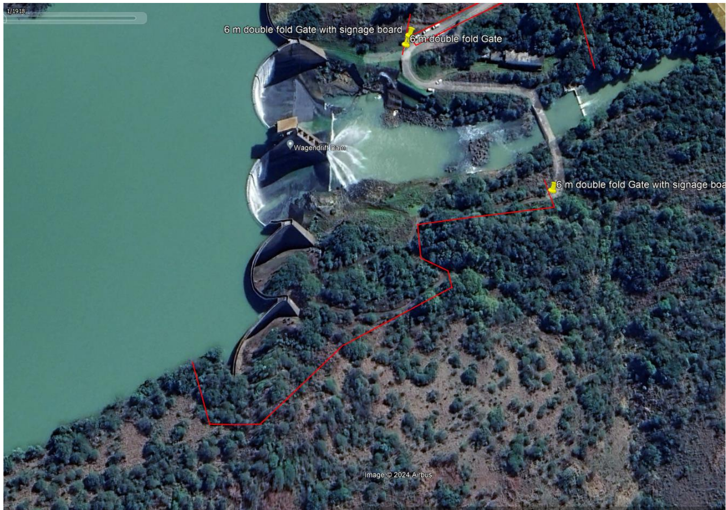
Wagendrift Dam right bank fence line in red
