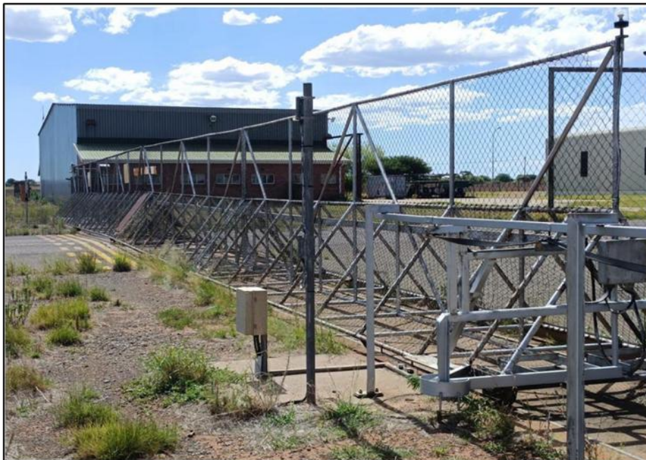
Figure 1: Bravo Taxiway Gate at Kimberley Airport
