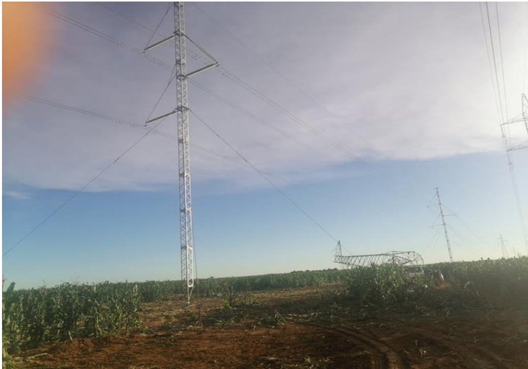
Figure 1.4: Two KEMA (ERS) towers installed
