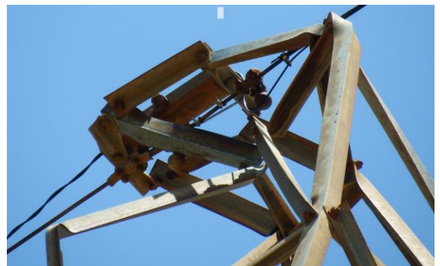
Figure 1.2: Tower 238 – Damaged Earthpeak
