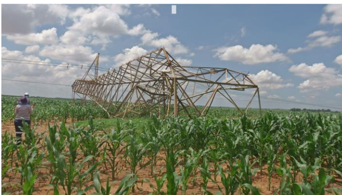
Figure 1.1: Tower 237 - Collapsed
