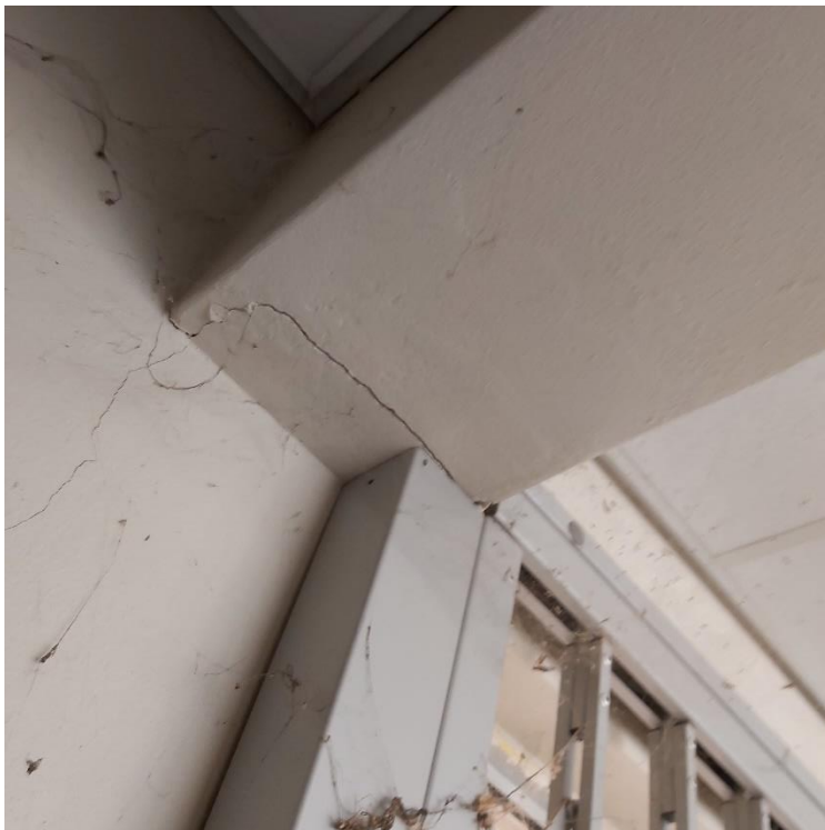
Figure 30 – Beam-to-Wall Interface of the RC Ring Beam of the Administration Building (internal)
