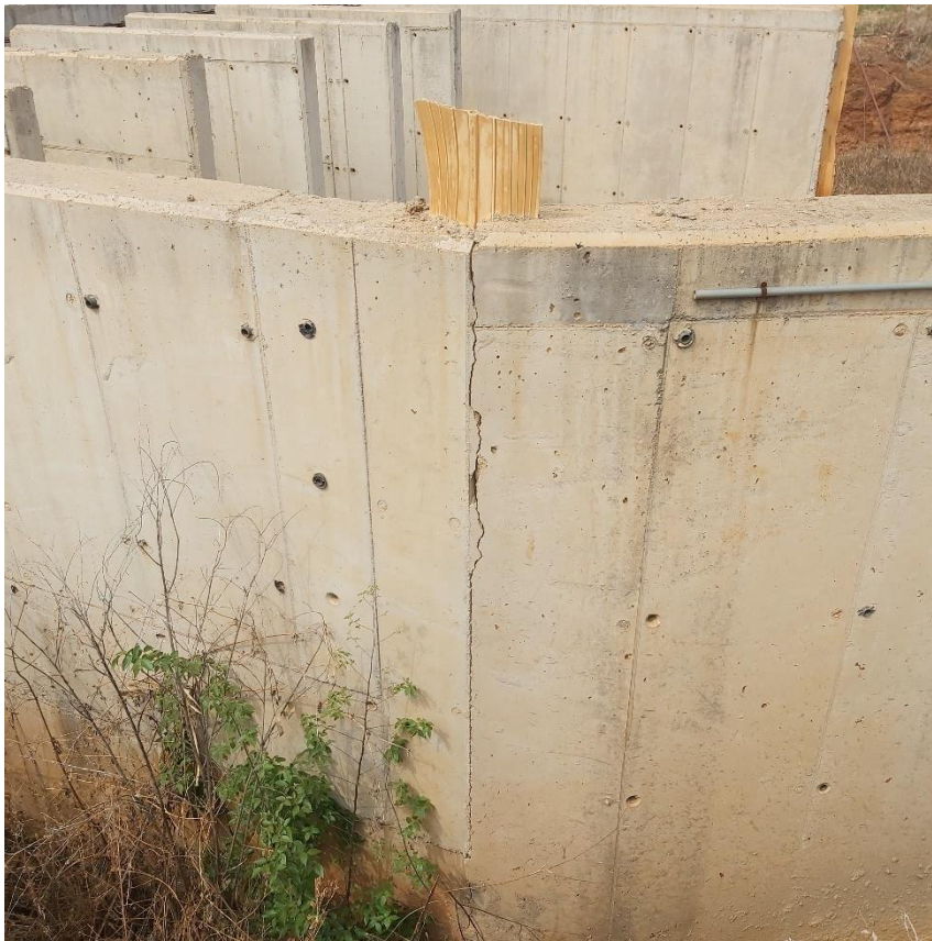
Figure 5 - Crack along a specified expansion joint on the RC Wall
