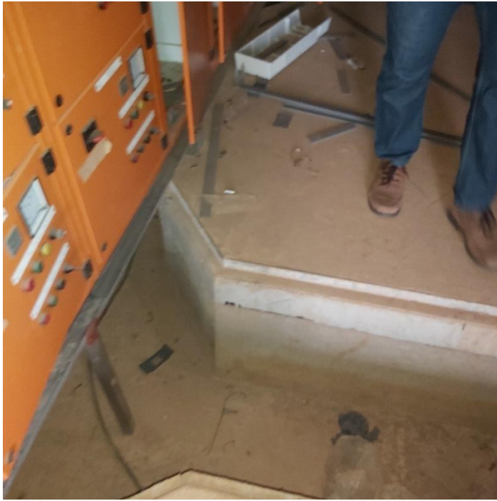
Figure 36 - MCC Building Surface Bed and Cable Trench
