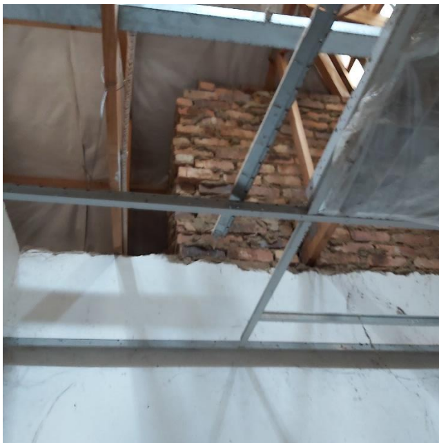
Figure 33 - Internal Firewall for the Administration Building
