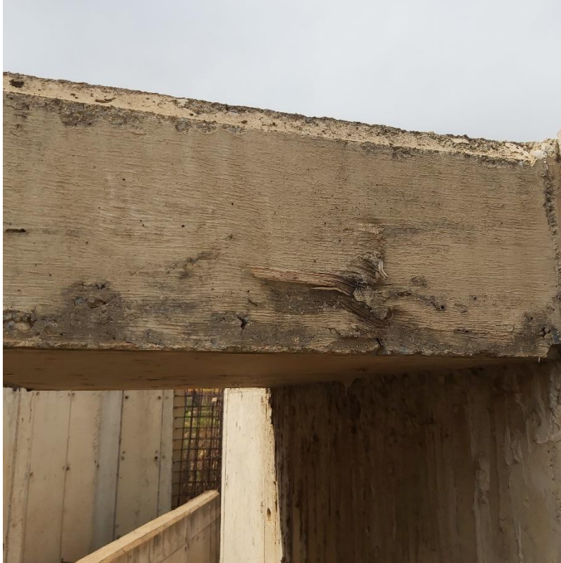
Figure 9 - Timber material cast into concrete within the platform suspended slabs
