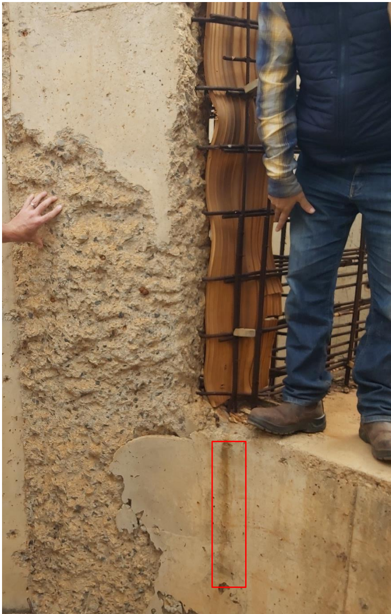
Figure 6 - Signs of concrete remedial works on the Jet Air Grit Trap Walls
