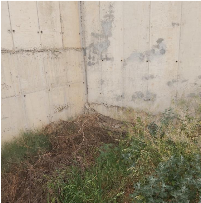
Figure 22 - Substandard Concrete Joints Observed on the Biological Reactor Reinforced Concrete Walls
