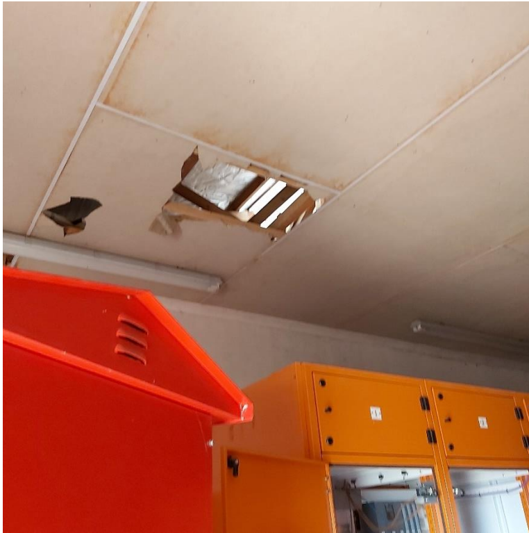
Figure 39 - Open Section on the Ceiling and Roof of the MCC Building
