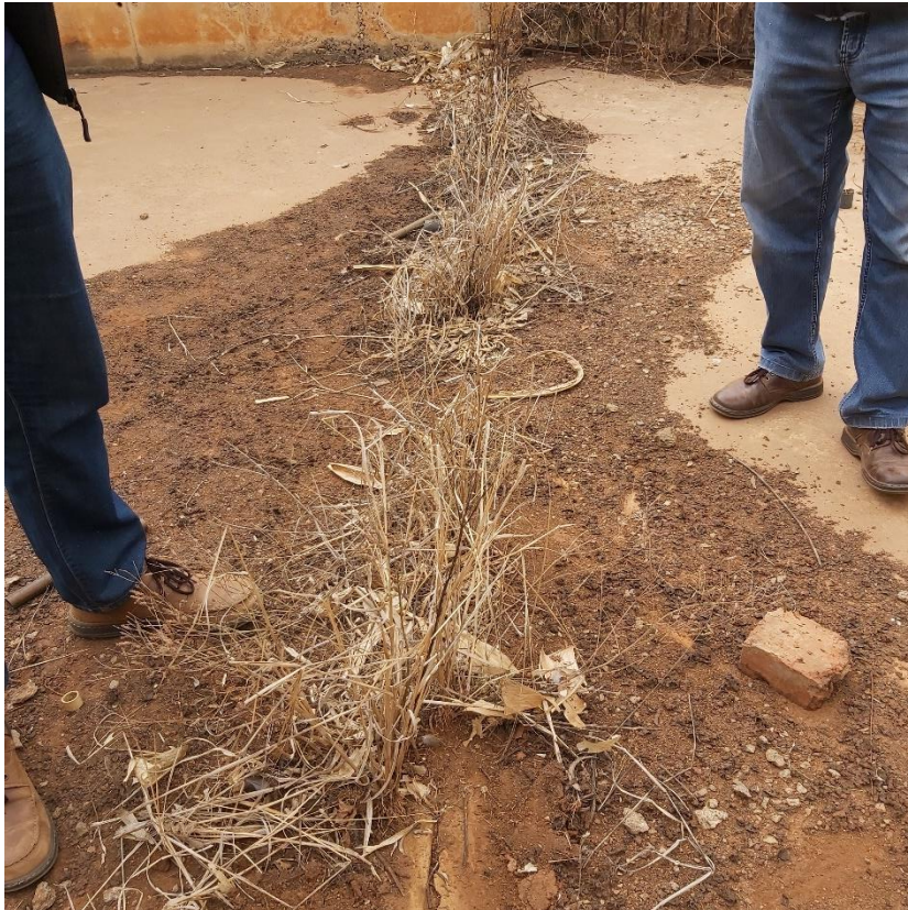
Figure 4 - Vegetation outgrowth through expansion joint on the surface bed
