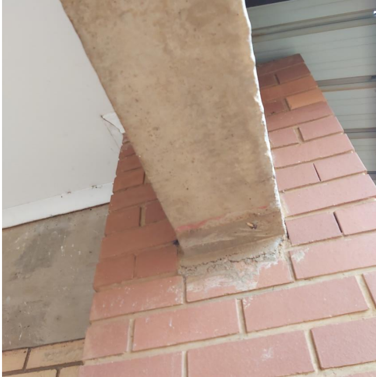
Figure 29 - Beam-to-Wall Interface of the RC Ring Beam of the Administration Building (external)
