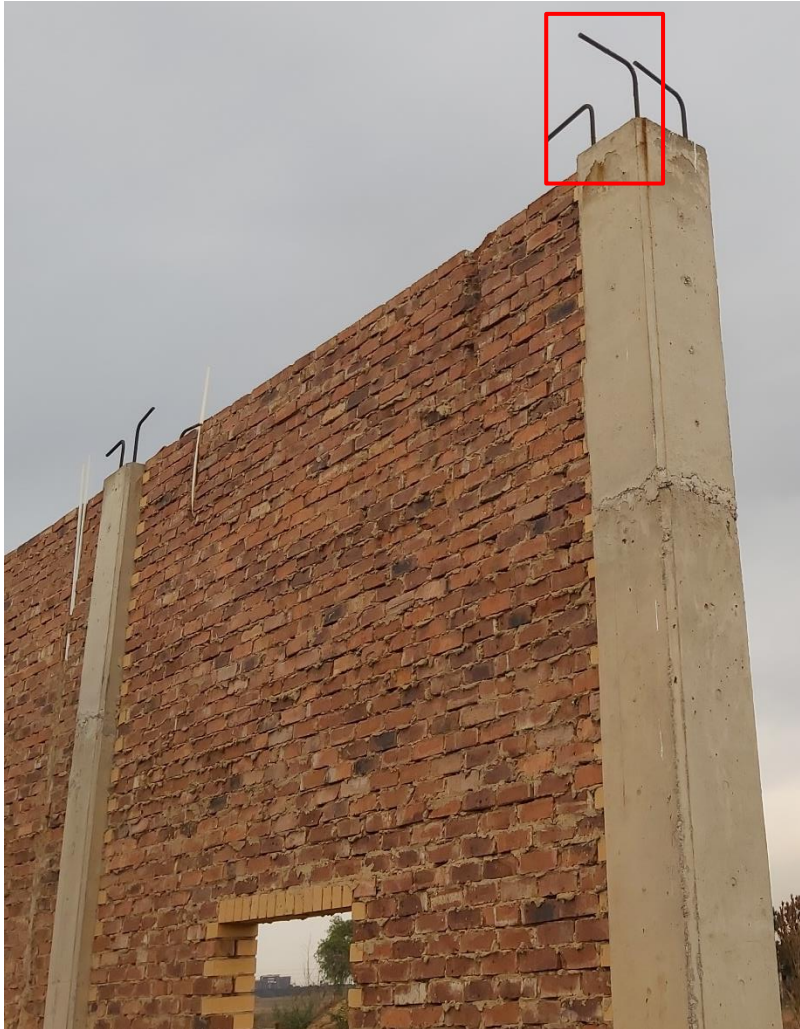
Figure 16 - Transfer rebars from column to 400mm x 400mm deep Ring Beam
