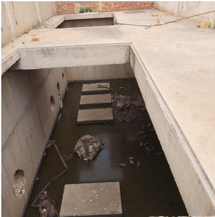
Figure 13 - Ponding water on the basement surface bed of the raw water pump station
