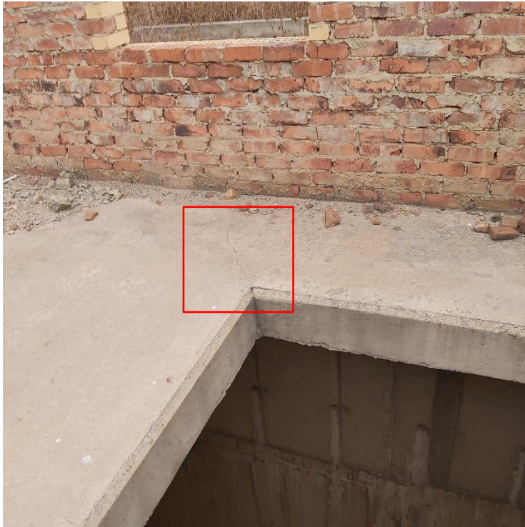
Figure 14 - Cracks propagating from the corners of open sections of the slab
