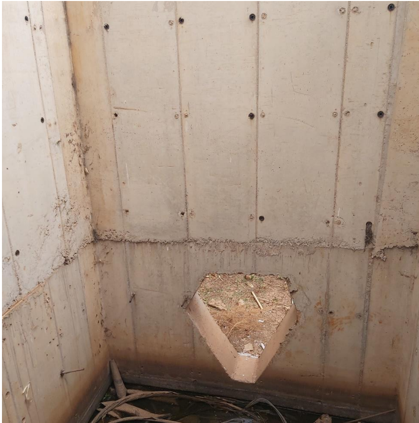
Figure 7 – Sub-standard wall casting and jointing observed around the perimeter of the structure
