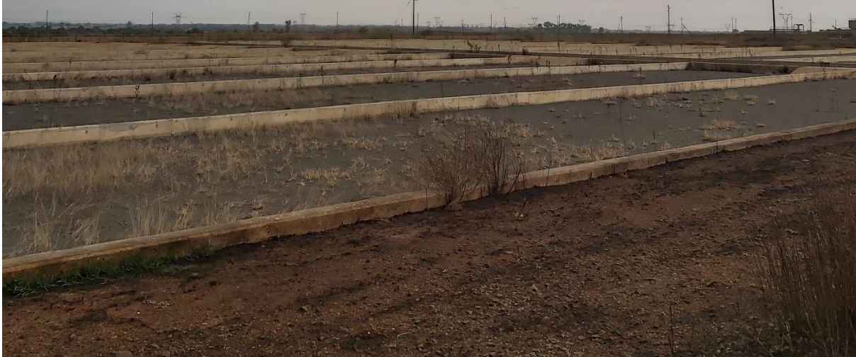
Figure 25 - Sludge Drying Bed
