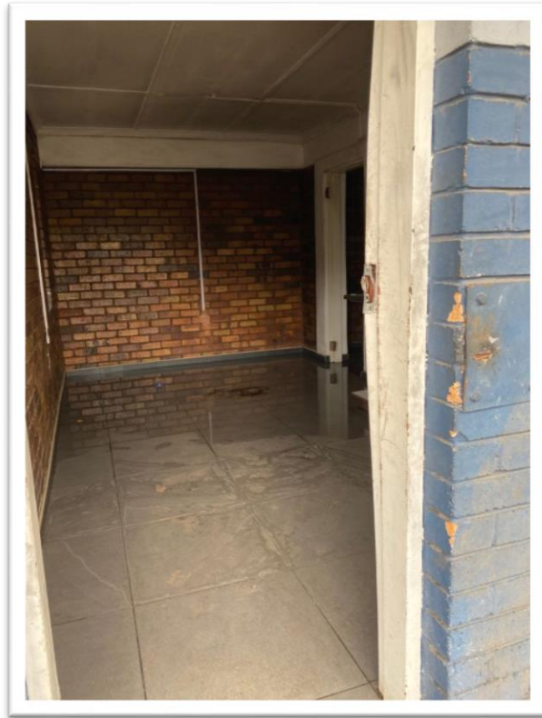
Inside the building.
