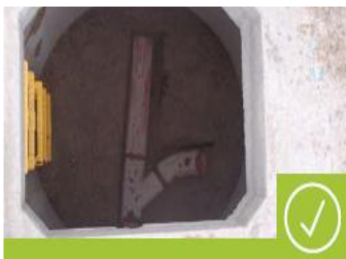
Example of a manhole benching
