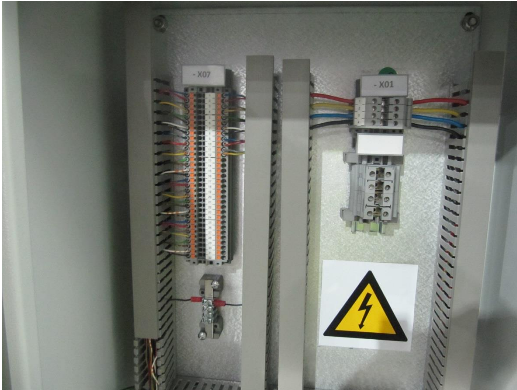
Figure 8: Typical Internal Layout of a Splitter Box
