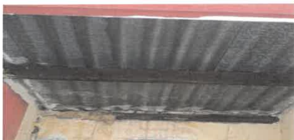
Figure 20: Picture of Roof Structure (Internal)
