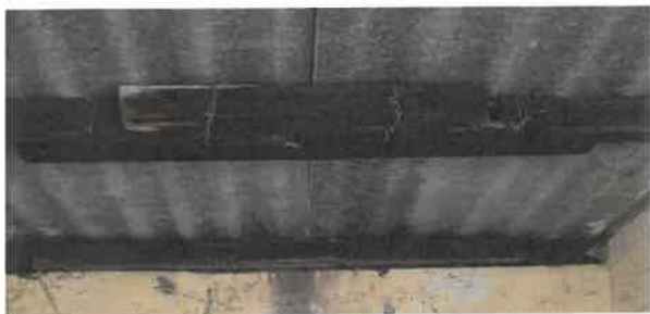
Figure 9: Picture of Roof Structure (Internal)
