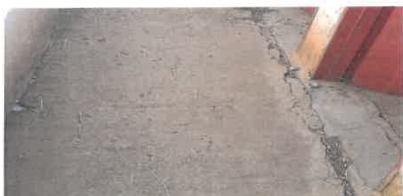
Figure 22: Picture of Internal Floor
