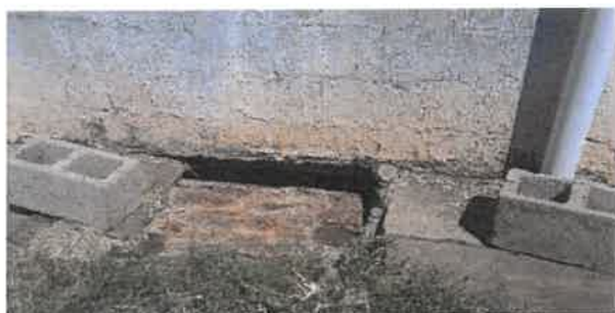
Figure 6: Pit Collapsing
