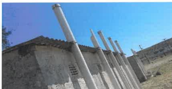
Figure 21: Picture of Roof (External)
