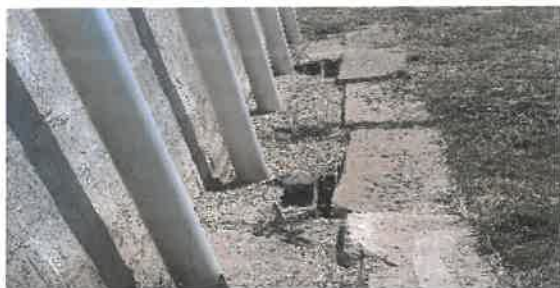
Figure 17: Pit Collapsing
