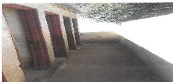
Figure 11: Picture of Internal Floor
