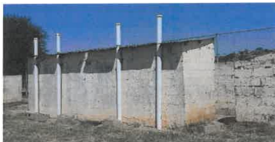
Figure 10: Picture of Roof (External)
