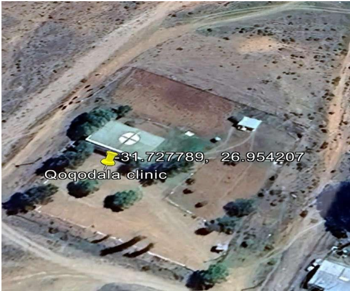
QOQODALA CLINIC AERIAL VIEW (SOURCE GOOGLE EARTH)
