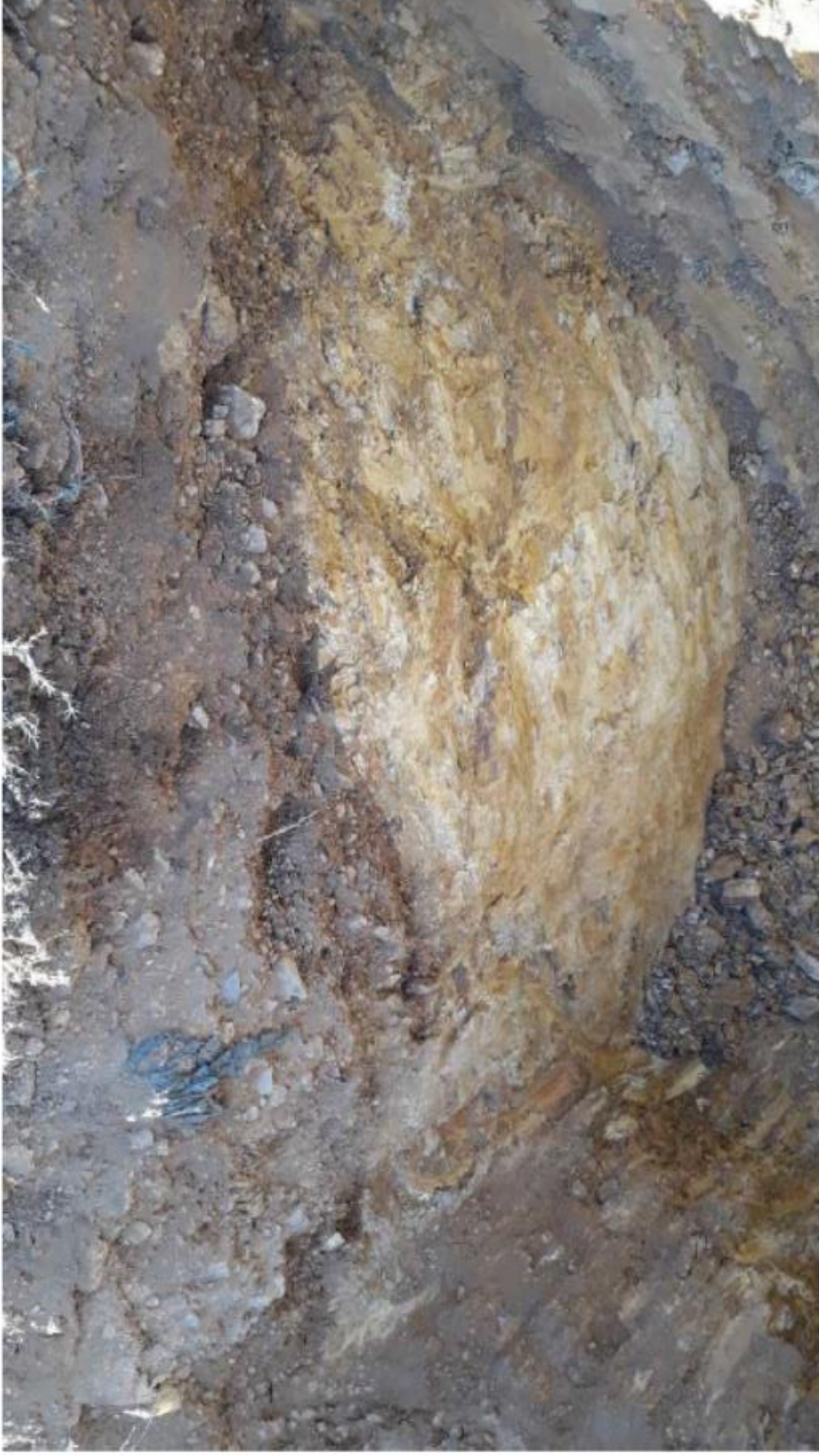
Photo 4 – View of typical trial hole profile comprising predominately weathered phyllites.
