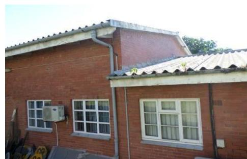
Remove asbestos roof and replace with new roof coverings.
