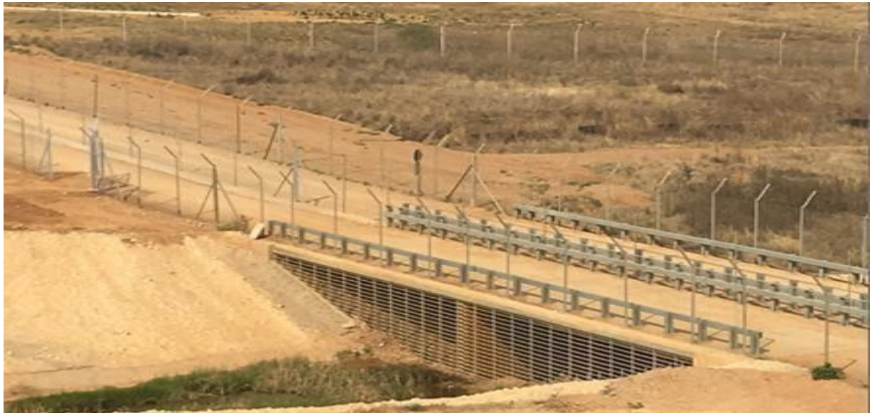
Figure 7: Security Grid Arrangement (Culvert/Bridge Crossing)
