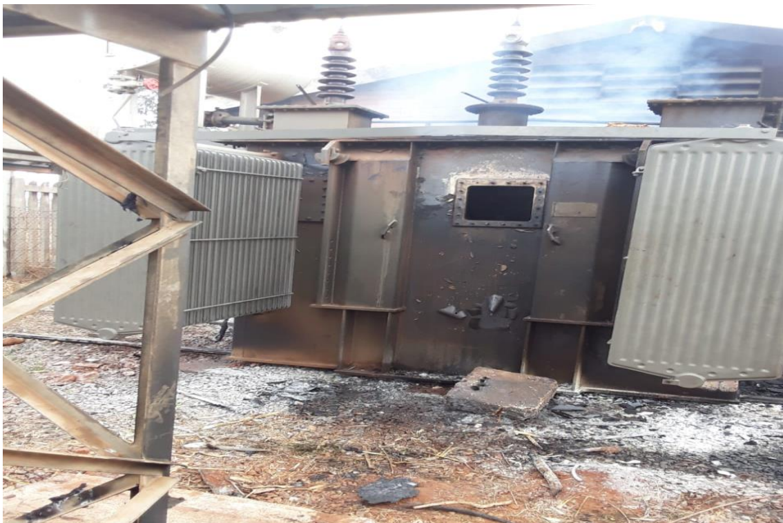
Figure 3: Main transformer vandalized
