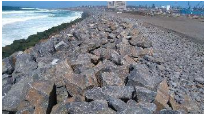
Figure 4: Foreshore Rock Protection
