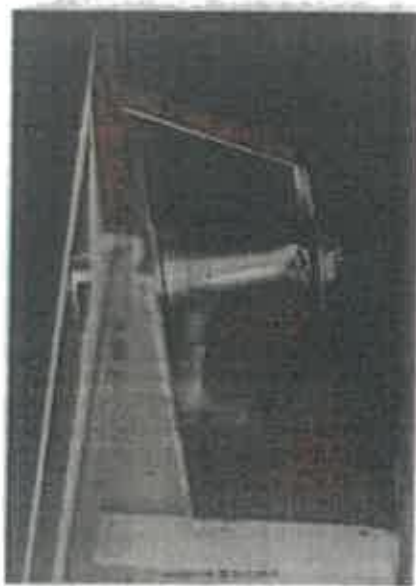
Factory fitted metered tap that runs for 8-15 seconds.
