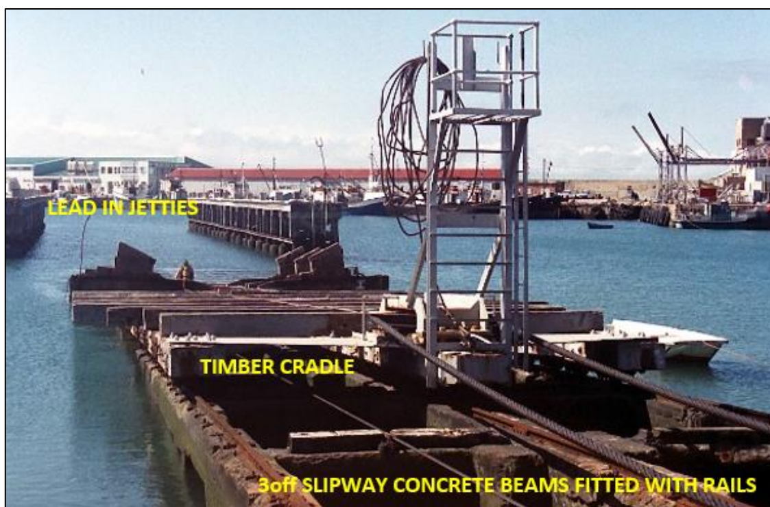
Figure 1: Existing slipway facility at the Port of Mossel Bay
