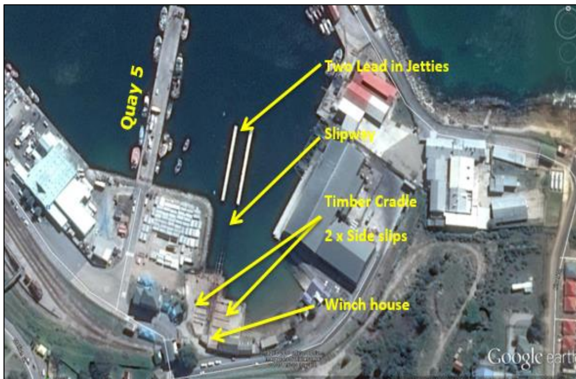
Figure 4: Location of the slipway at the Port of Mossel Bay
