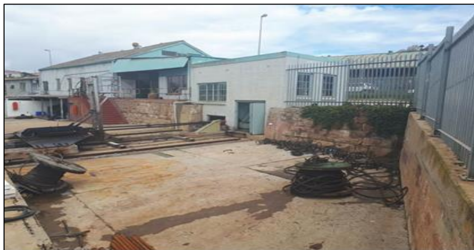
Figure 3: Slipway operations building
