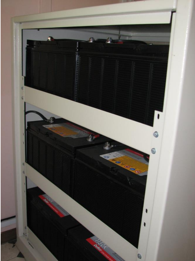
Figure 5: Library UPS, Batteries
