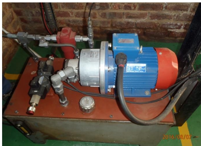
Pongolapoort Dam: 3800mm Outlet Line: Hydraulic Power Pac
