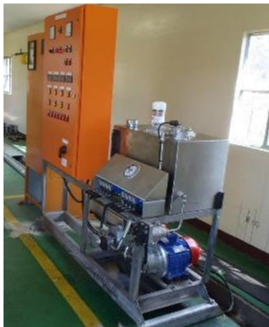
Pongolapoort dam: Canal outlet Hydraulic Power Pack
