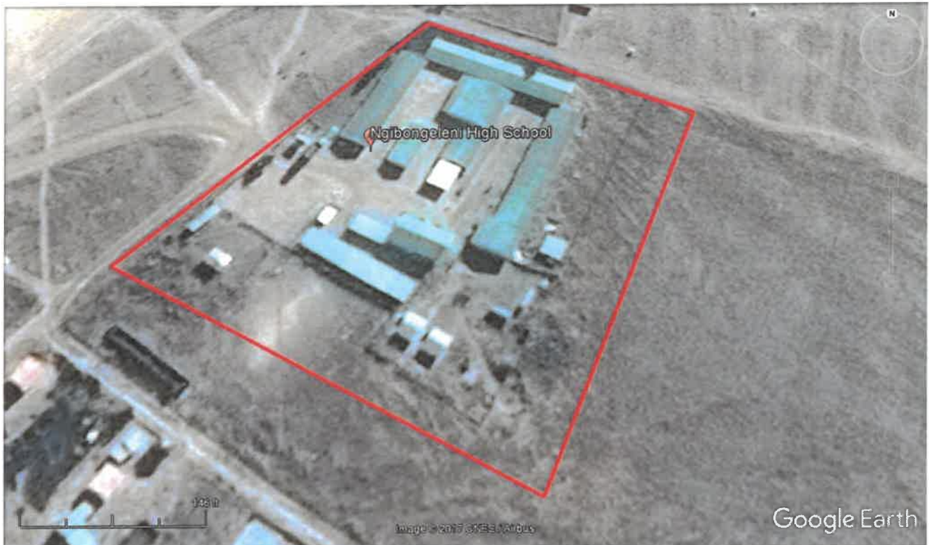
Figure 1: Ngibongeleni High School (sourced from Google Earth).
