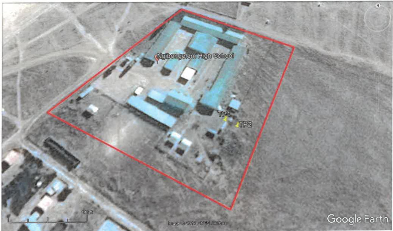
Figure 3: Test Pit Positions (sourced from Google Earth)
