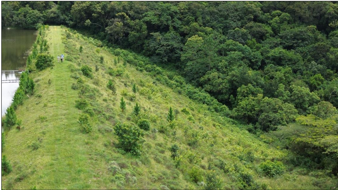
Figure 1: Overview of dam wall
