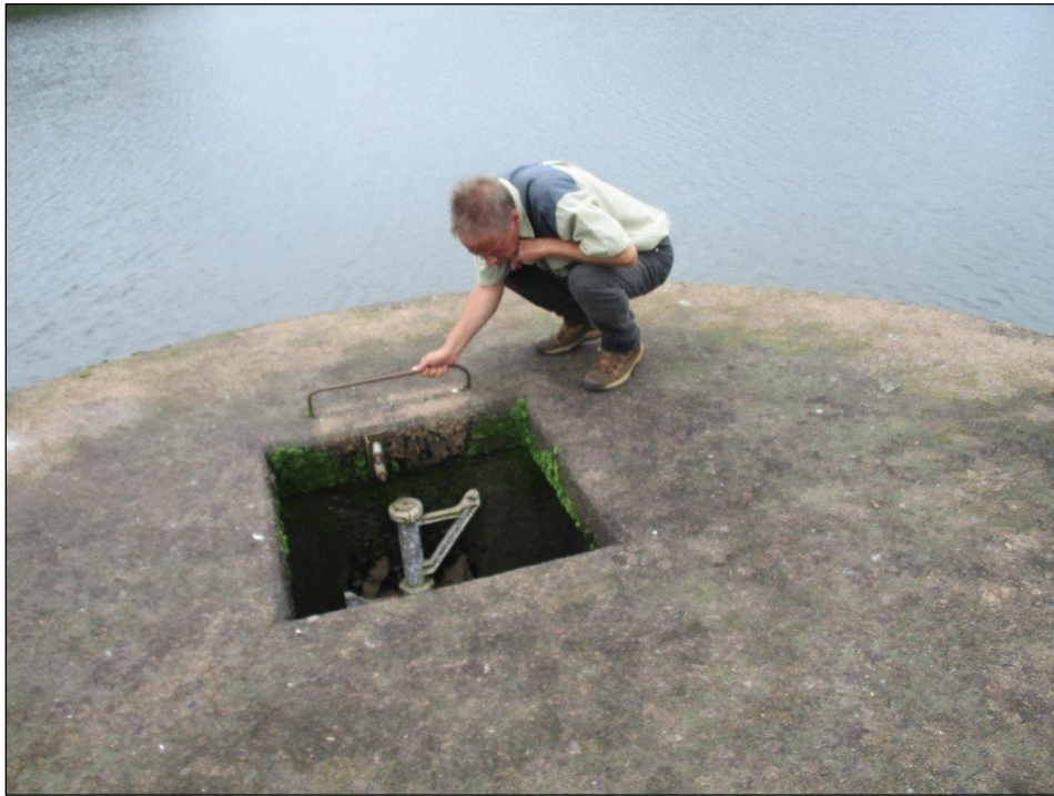
Figure 5: Access opening on top of intake tower
