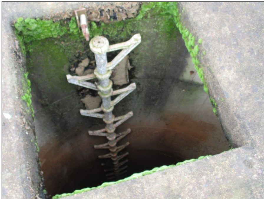
Figure 8: Current ladder inside tower
