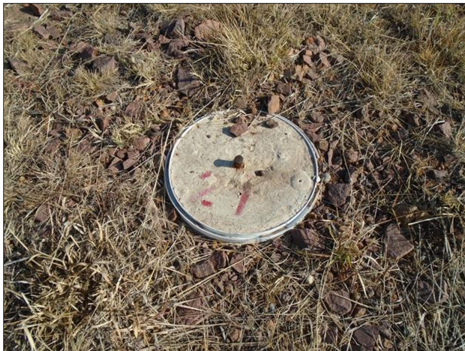
Figure 3: Settlement beacon typical example
