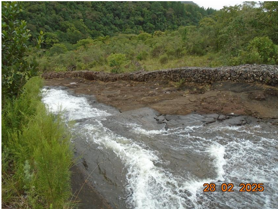
Figure 4: View of gabion side wall
