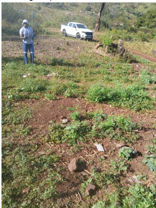
Figure 14: Image of DCP Test at position X 6
