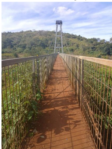
Figure 3: Access bridge to the Maqhashiya Primary School
