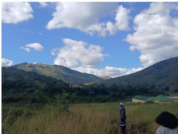
Figure 9: Image of DCP Test at position X_3
