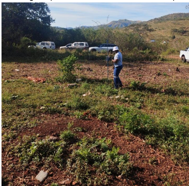
Figure 12: Image of DCP Test at position X 4
