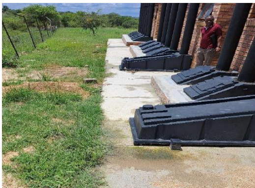
Pit toilets saturated by groundwater
