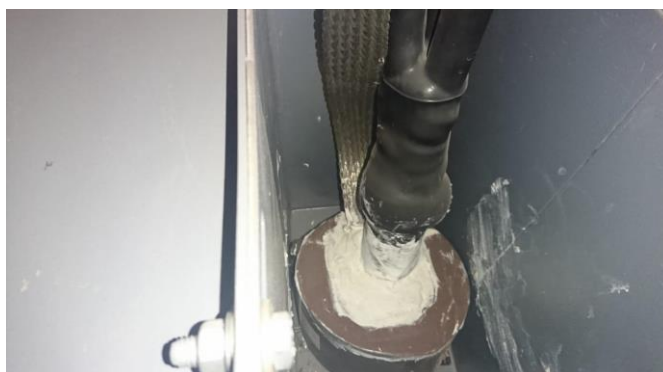
Figure 18: Example of INCORRECTLY installed core balance CT
