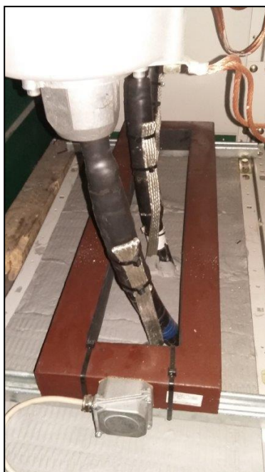
Figure 17: Examples of correctly installed core balance CTs
