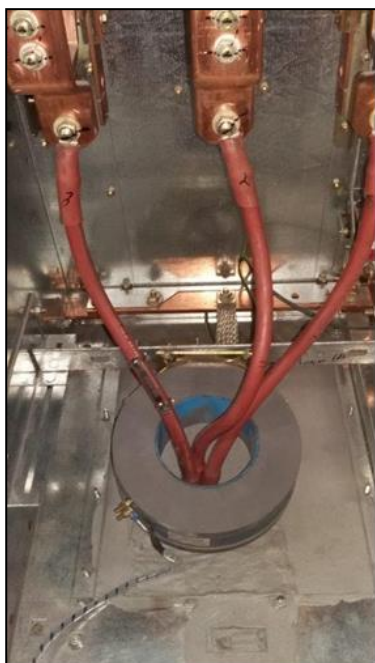
Figure 17: Examples of correctly installed core balance CTs
