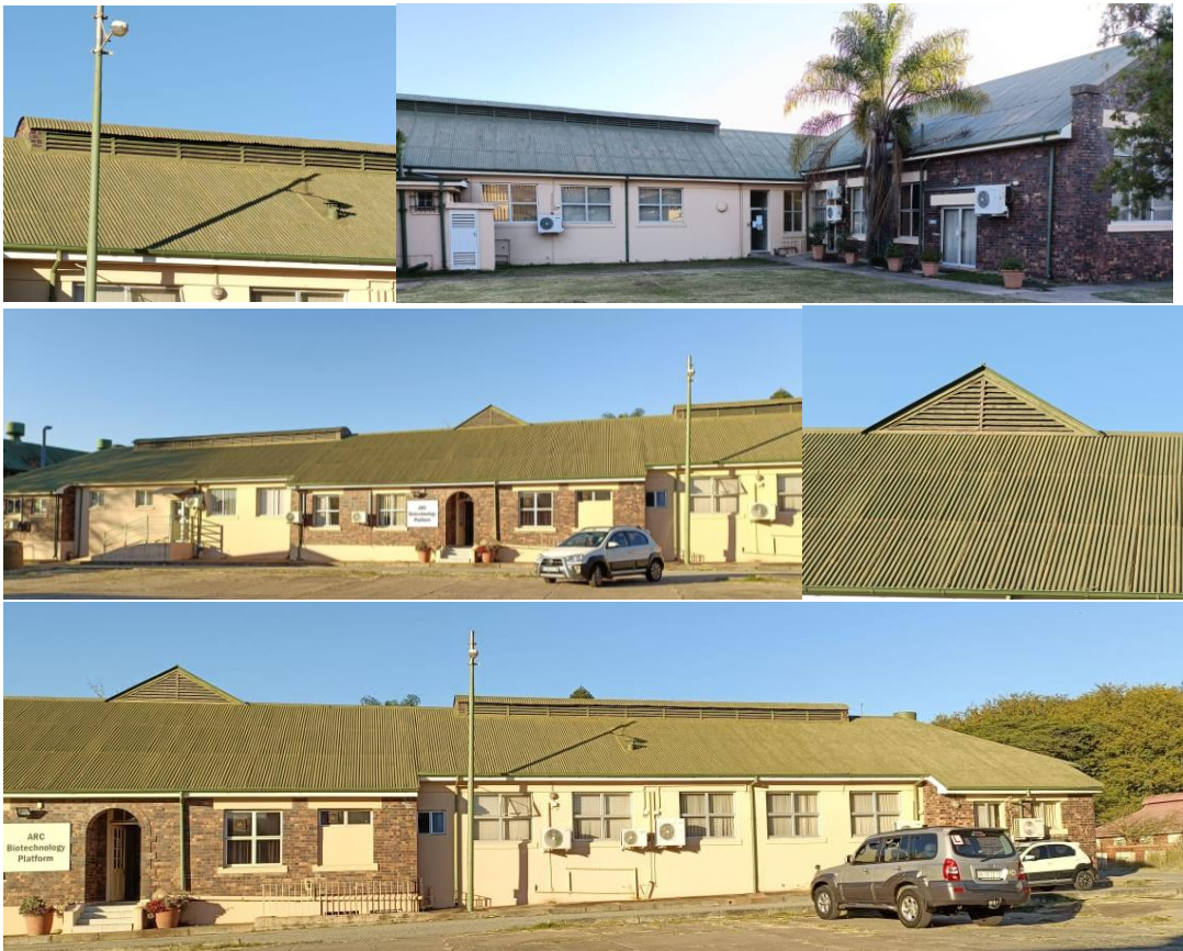
Figure 1. Biotechnology Platform building's roof, wooden louvres, gutters, downpipes and Fasi boards showing that will require cool surface prep and painting.
