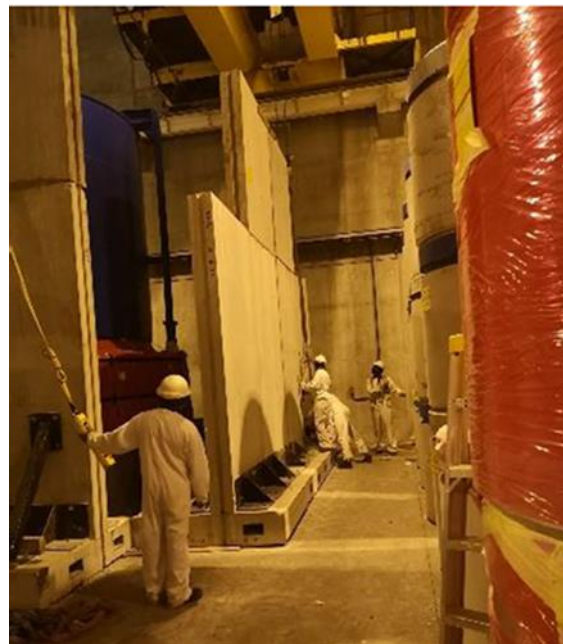
Figure 5 : Unit 2 showing extra height extra-high concrete panel walls, being installed
