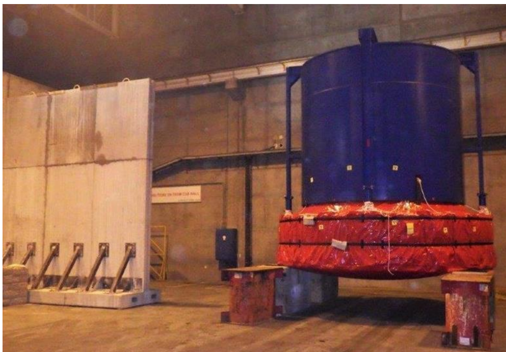
Figure 2: Unit 2 RPVCH mounted on concrete blocks at LLW building
